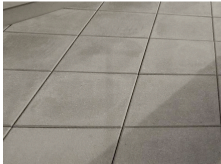
A SAND-SET PRECAST PAVERS
