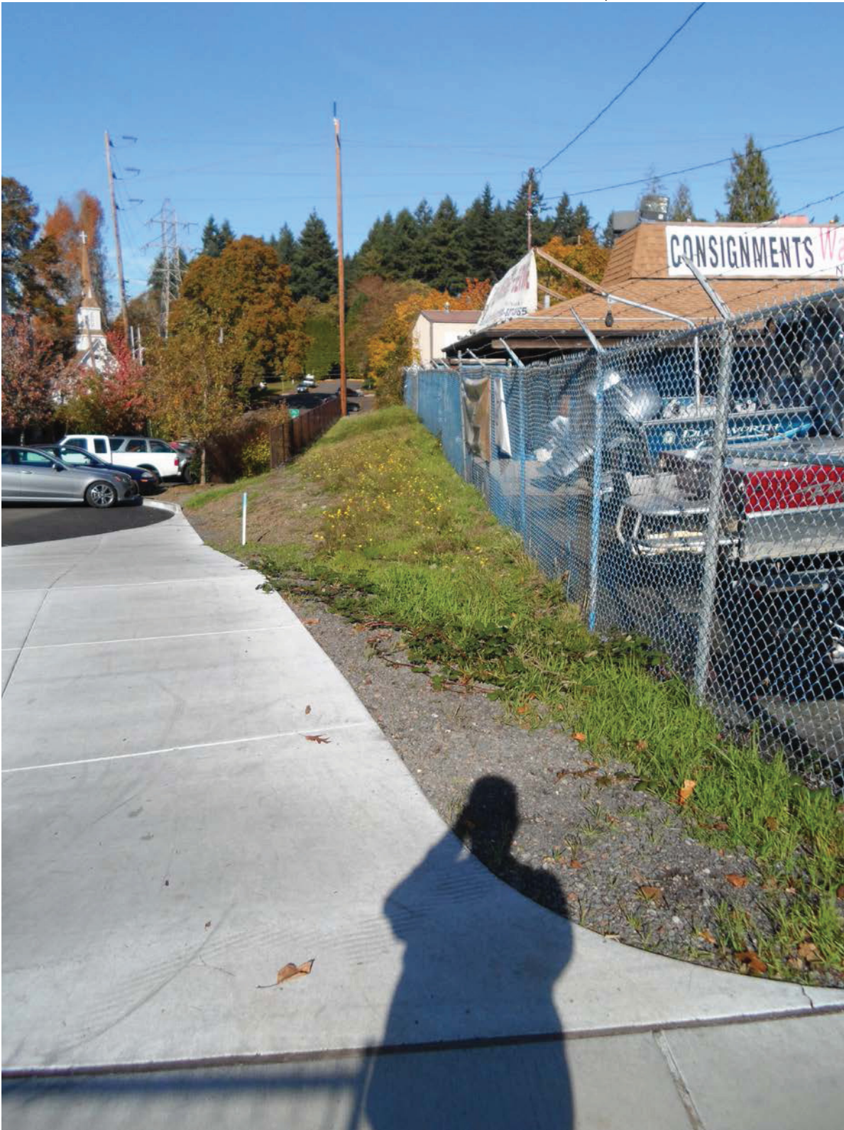
Looking north at new bike ramp and STV area.
