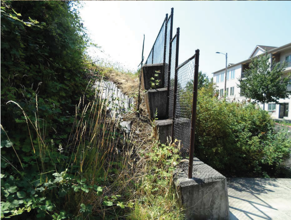
Looking south from Spokane Street at retaining wall.
