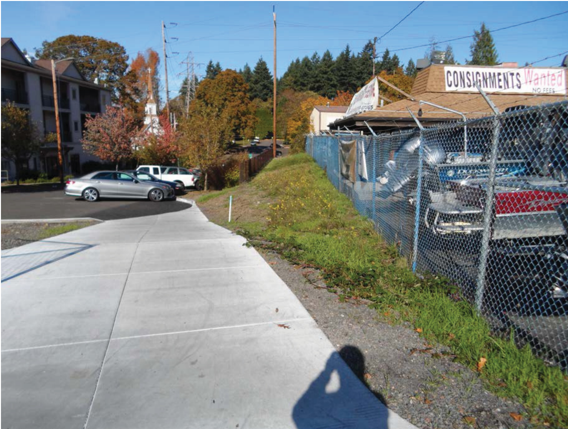
Looking north at new bike ramp and STV area.
