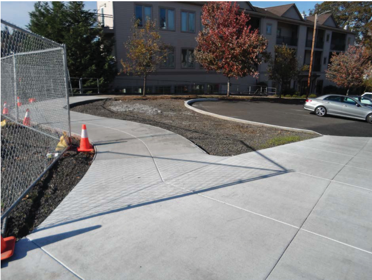
Looking northwest from Tacoma St. at new cul-de-sac.
