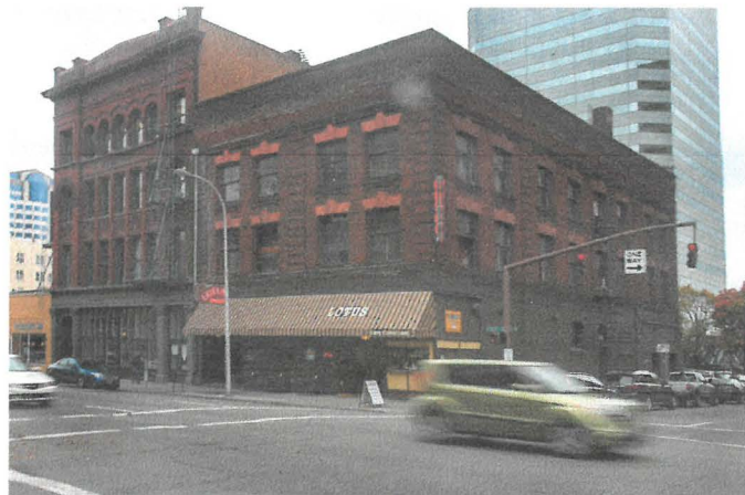
The Ancient Order of United Workmen Temple (top) and Hotel Albion (bottom) were removed from the Historic Resource Inventory November 5 to make way for demolition.
