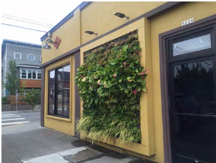
Example of a vegetated green wall
