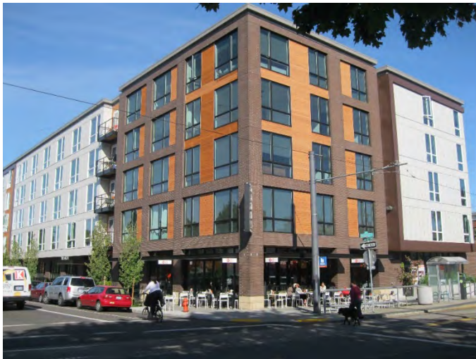
As Portland grows, development in the commercial /mixed use zones will meet an increasing share of the city’s housing and employment needs.
