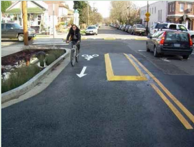
Curb Extension with Island Semi-Diverter: blocks vehicle entry to a street by closing off the parking lane on the entry street. This semi-diverter includes a bio-swale as part of the design.
