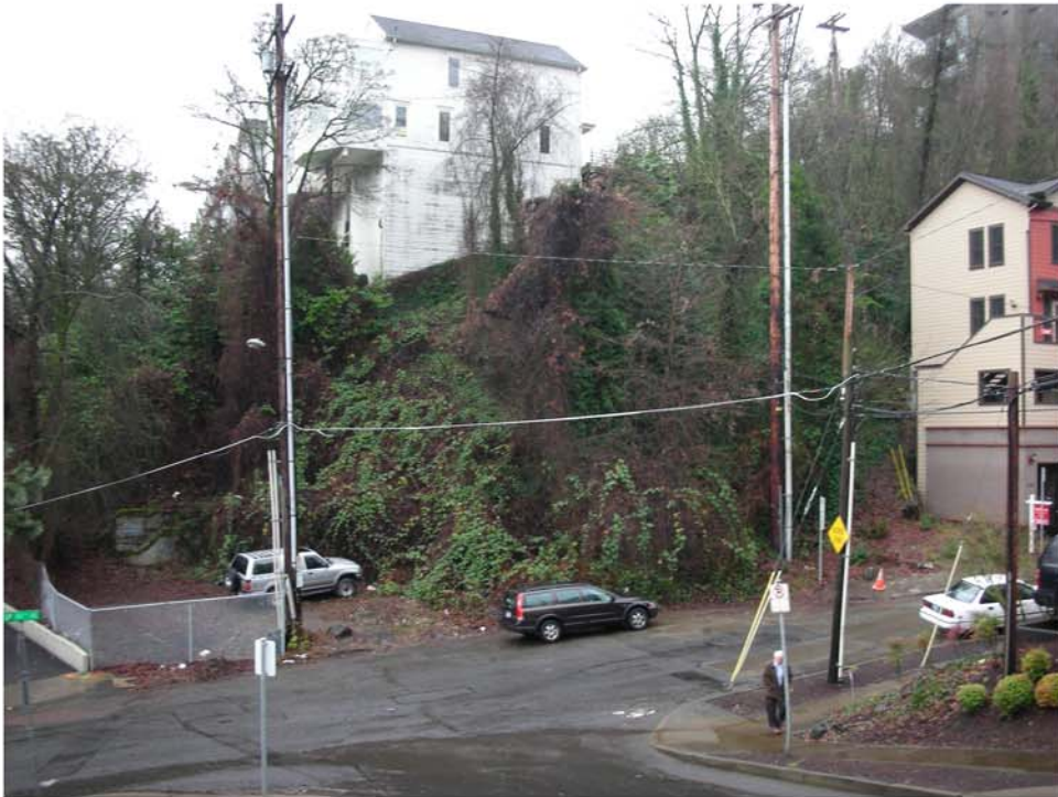
Site Observed from Mill st., looking east
