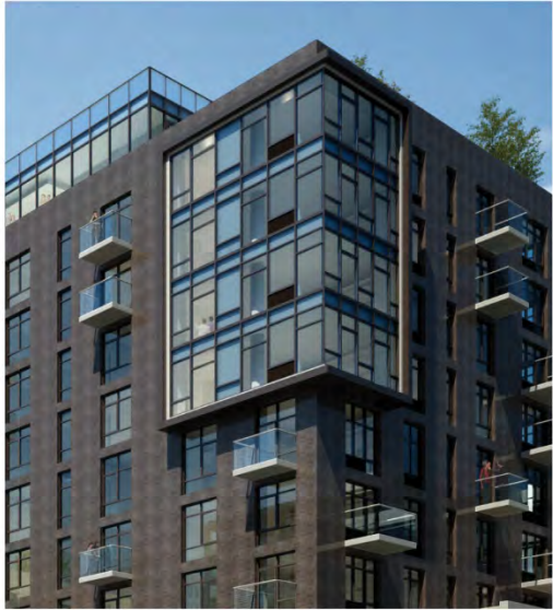
IMAGE OF SOUTHWEST CORNER CURTAIN WALL
