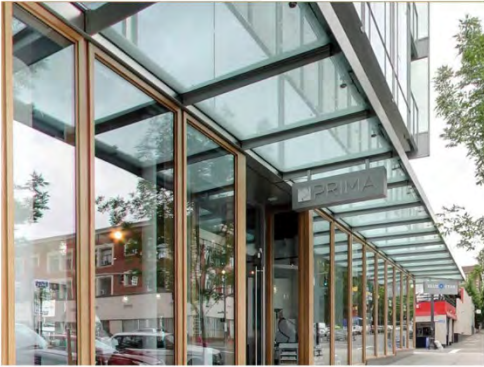
REPRESENTATIVE IMAGE OF STEEL GLASS CANOPY
