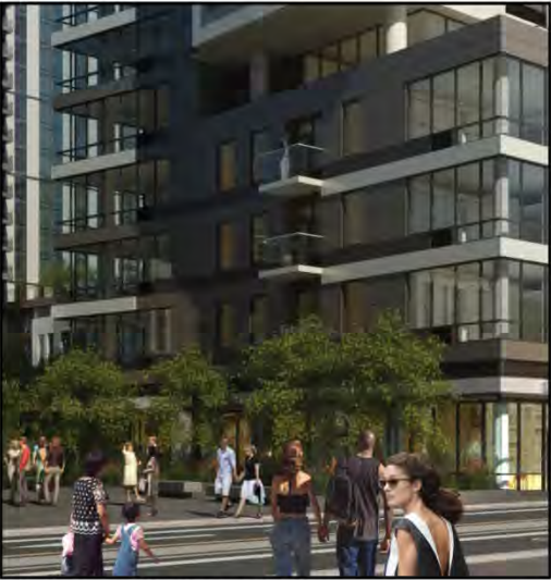
IMAGE OF PODIUM AT NW CORNER
