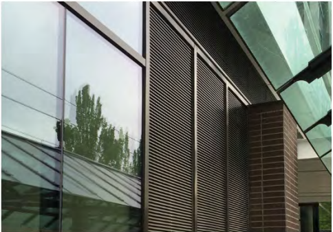
REPRESENTATIVE IMAGE OF METAL LOUVER AT GROUND FLOOR
