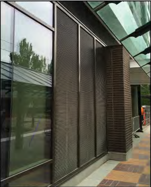
REPRESENTATIVE IMAGE OF METAL LOUVERS AT GROUND FLOOR
