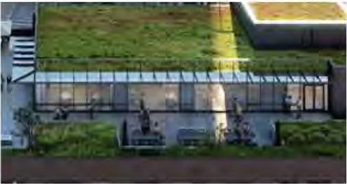
IMAGE OF ROOF CURTAIN WALL
