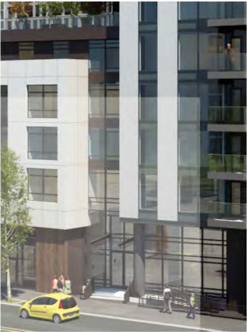
VIEW OF PASS-THROUGH LOBBY - NE OREGON ST
