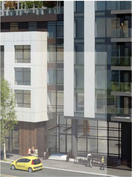
VIEW OF PASS-THROUGH LOBBY - NE OREGON ST
