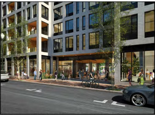
IMAGE OF PASS THROUGH LOBBY FROM NORTH
