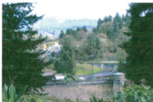
Figure 22: Photo of Reservoir 4 from above showing the existing Reservoir 4 and the existing Reservoir 4 Dam. The view is from above at Sherwood Blvd. - EXISTING
