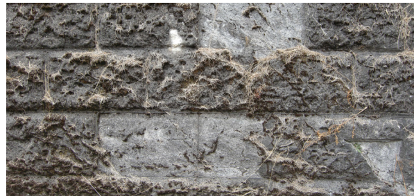
Figure 29: Reservoir 3, spalled faces of Ransome concrete at the northwest wall
