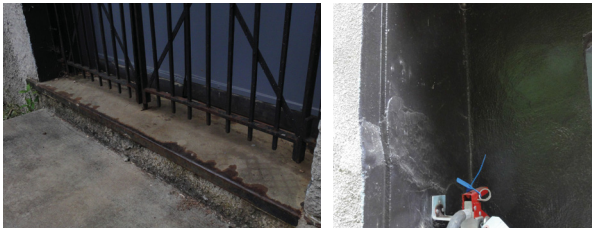
Figure 67: L- South door, original cast iron sill; R- East door, jog in frame
