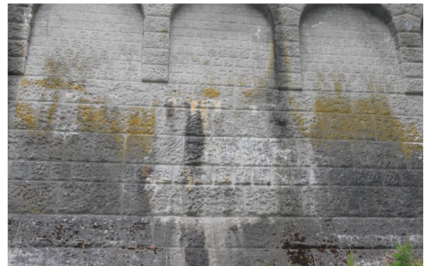
Figure 22: Reservoir 3, dam face water leaking from crack with efflorescence
