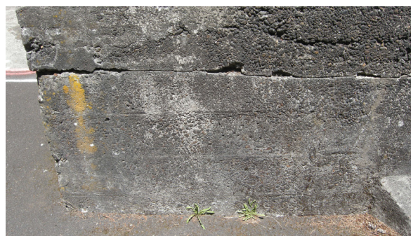
Figure 57: Continuous crack along slab edge
