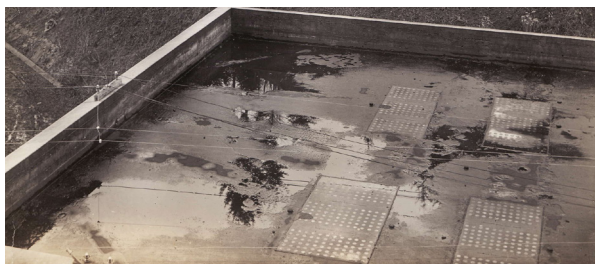
Figure 60: Pump House 1, original Ransome Patent Lights
