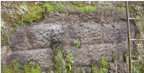
Figure 31: Reservoir 4, retaining wall, water saturated and biological growth
