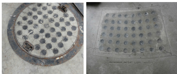
Figure 59: Gatehouse 4, original Ransome Patent Lights
