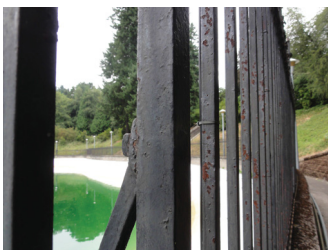
Figure 39: Corrosion of ironwork and peeling paint
