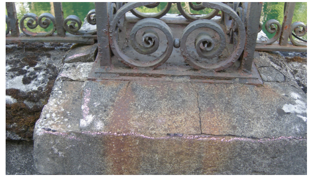
Figure 15: Reservoir 3, concrete delamination at the parapet wall column
