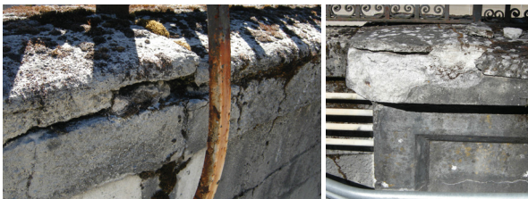
Figure 21: Reservoir 4, dam parapet coping delaminated
