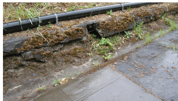
Figure 35: Gutter damage and exposed reinforcing
