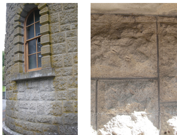
Figure 43: Biological growth; Repetitive horizontal cracks
