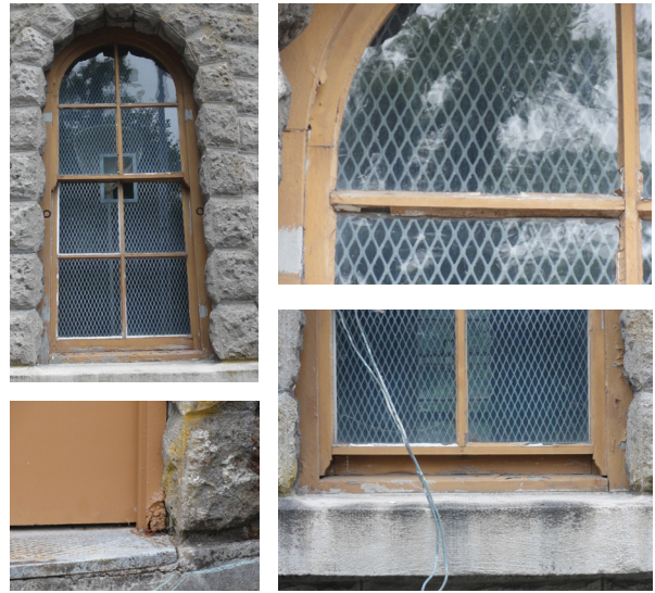
Figure 65: Gatehouse 4 door corrosion, window sealant deterioration, and peeling paint
