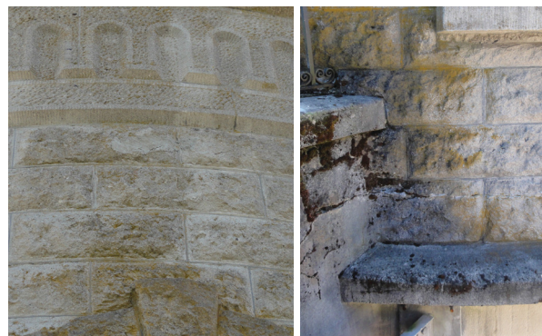
Figure 47: Staining and previous repairs above east door; Staining and continuous crack
