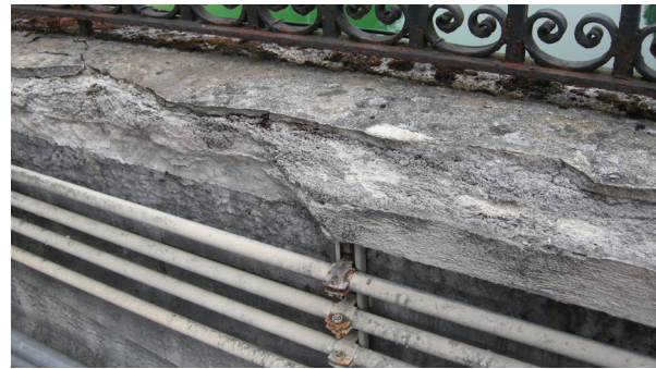
Figure 18: Broken coping on the dam parapet at Reservoir 3 :2013
