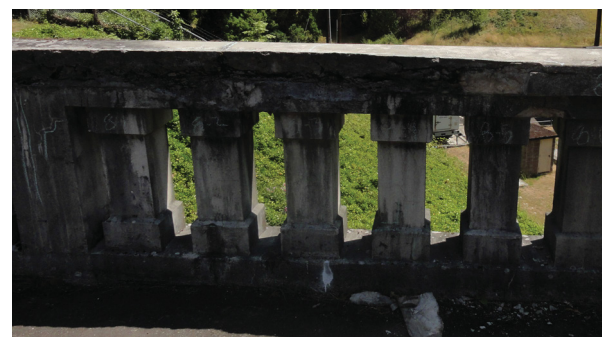
Figure 27: Reservoir 4, baluster delaminated and broken coping
