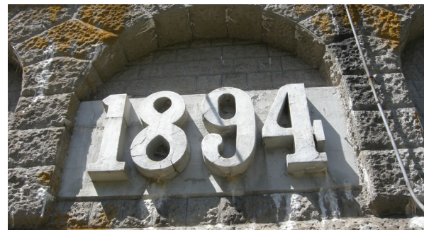
Figure 25: Reservoir 4, 1894 icon, cracks, biological growth, efflorescence
