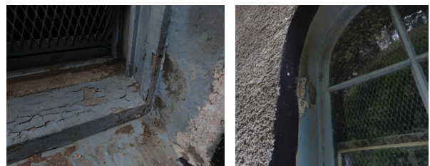
Figure 66: Peeling paint on south east window of Pump House 1
