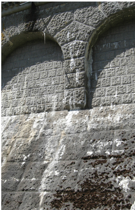
Figure 26: Reservoir 4, efflorescence, continuous crack, and staining on dam face
