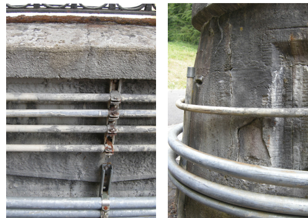
Figure 19: L- Finish and discoloration ; R - Large cracks around southwest corner
