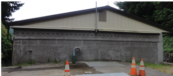
Figure 51: North elevation; Stuccoed window openings, horizontal cracks
