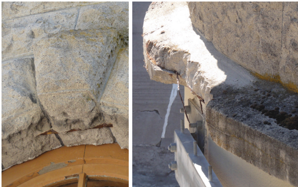
Figure 48: Exposed reinforcing at southeast window surround; Broken water-table base
