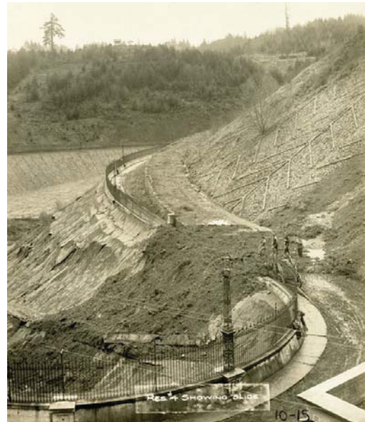
Figure 5. Early landslide damage to Reservoir 4
