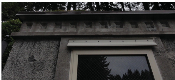
Figure 54: Stucco delamination; horizontal crack along cornice
