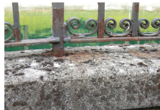
Figure 40: Fence connection with concrete parapet wall, welded connections
