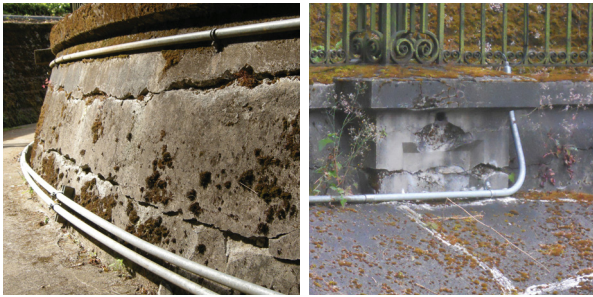
Figure 17: Large horizontal cracks at the southwest corner of Reservoir 4
