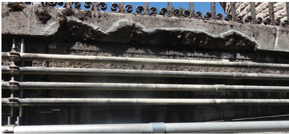
Figure 20: Reservoir 4, dam parapet coping delaminated
