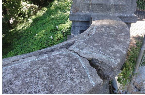
Figure 24: Reservoir 3, Large broken segment of the baluster rail
