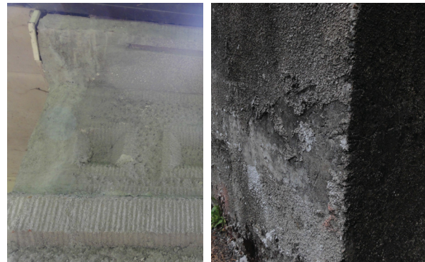
Figure 53: Stucco delaminating
