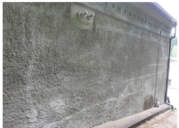
Figure 50: West elevation; previous repairs to multiple horizontal cracks
