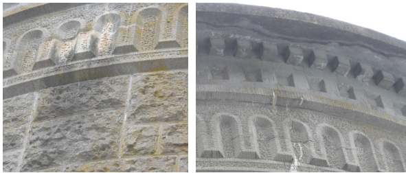
Figure 44: Crack along the frieze with staining and efflorescence
