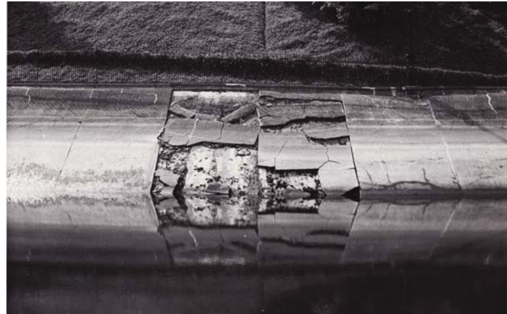
Figure 8. Photo of reservoir basin deterioration due to aging and slide movement
