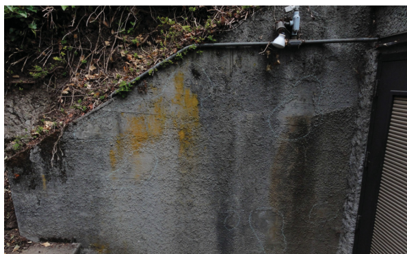
Figure 55: Delamination of stucco; biological growth; previous repair along door
