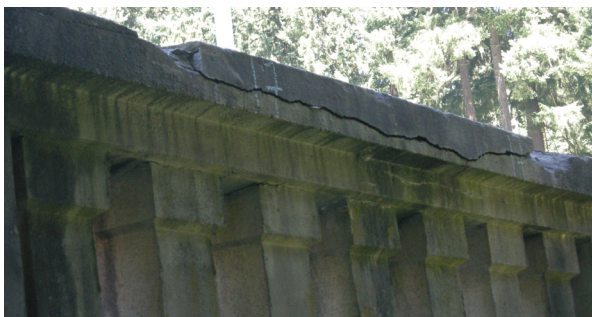
Figure 23: Reservoir 3, broken segment of the baluster coping
