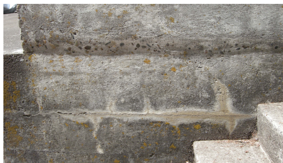
Figure 56: Crack and efflorescence
