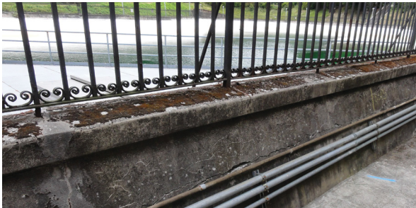
Figure 14: Reservoir 3, parapet wall deficiencies
