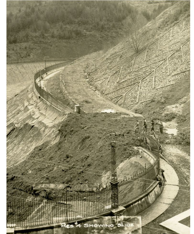
Figure 13. 1897 Landslide damage to Reservoir 4
