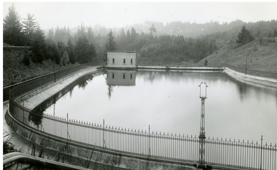
Figure 3. View of Reservoir 3 and Gate House 3 from the Grand Stairway, c. 1912
