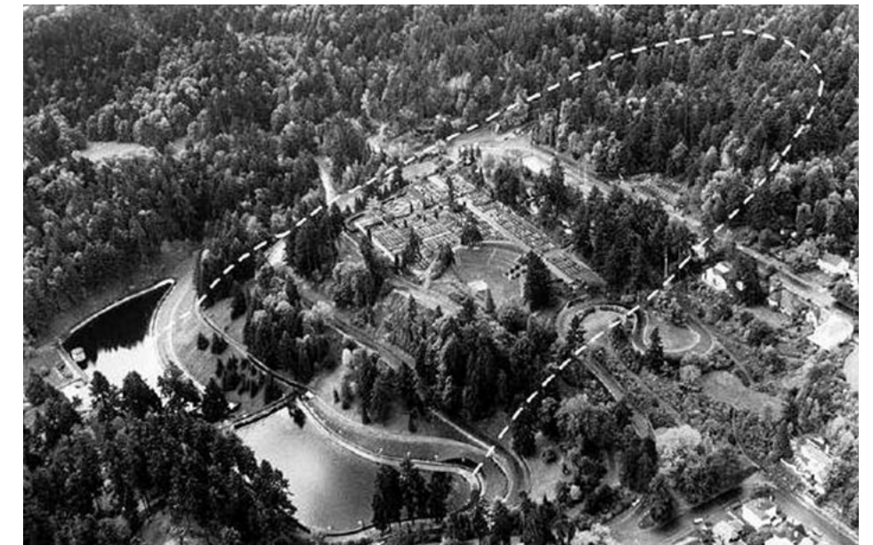
Figure 11. Historic photo of landslide zone, the Rose Garden, and the reservoirs
