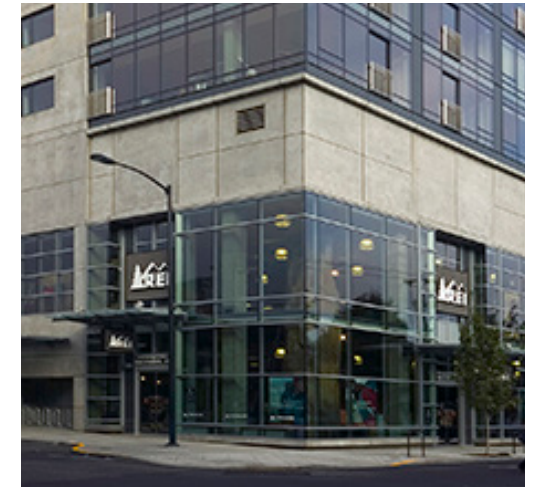
REPRESENTATIVE IMAGE OF FRAMED CURTAIN WALL
