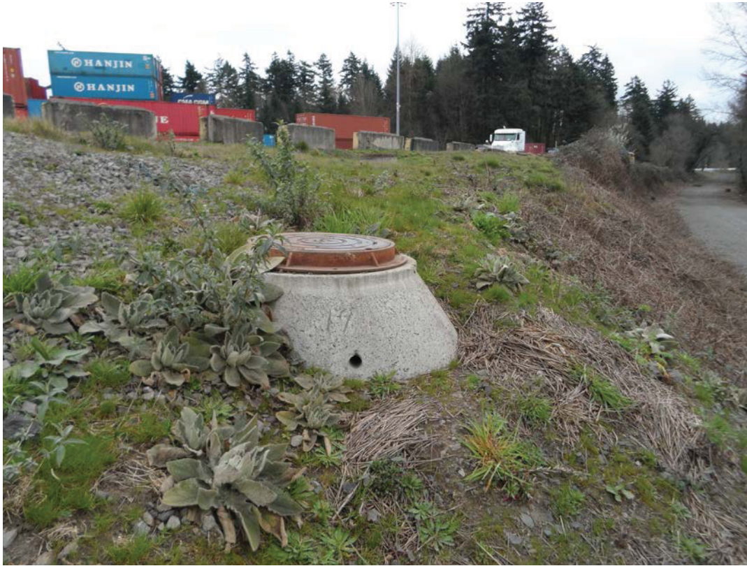
Figure 3: Looking easterly at storm sewer manhole in hillside portion of right-of-way.
