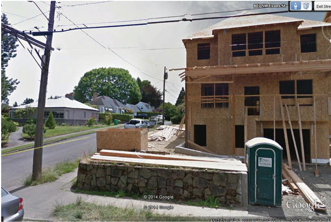
Scale and character of new infill is not compatible with existing home stock. This home dwarfs its neighbors.
