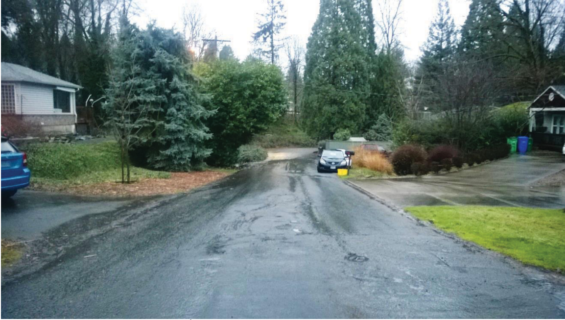
SW 14 th Avenue, facing north at SW Hume Street.
