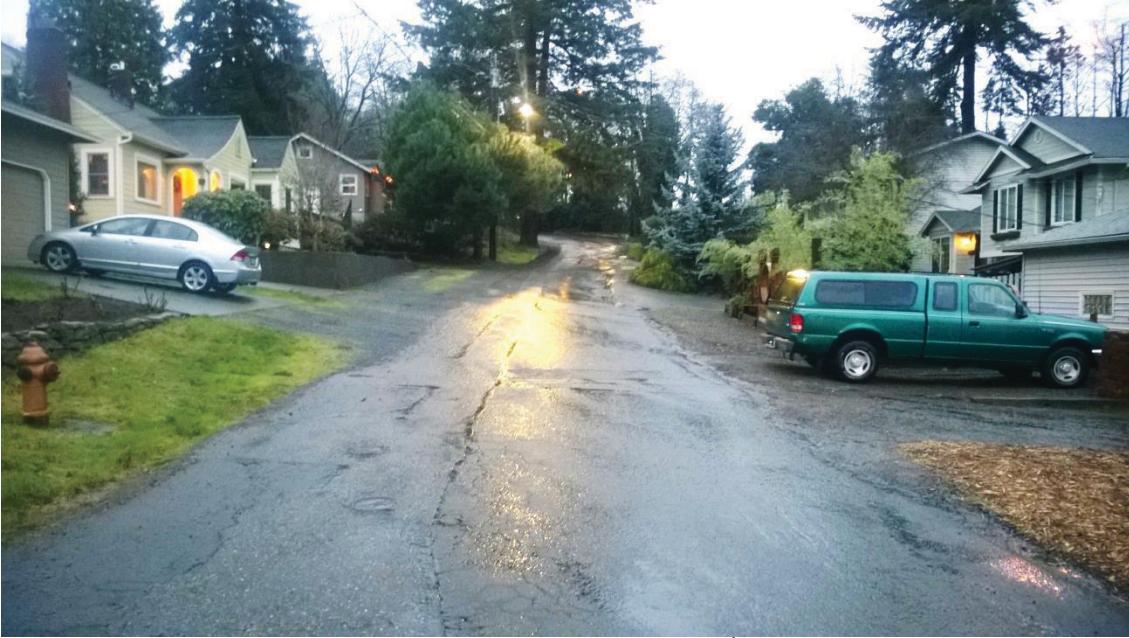
SW Hume Street, facing west at SW 14 th Avenue
