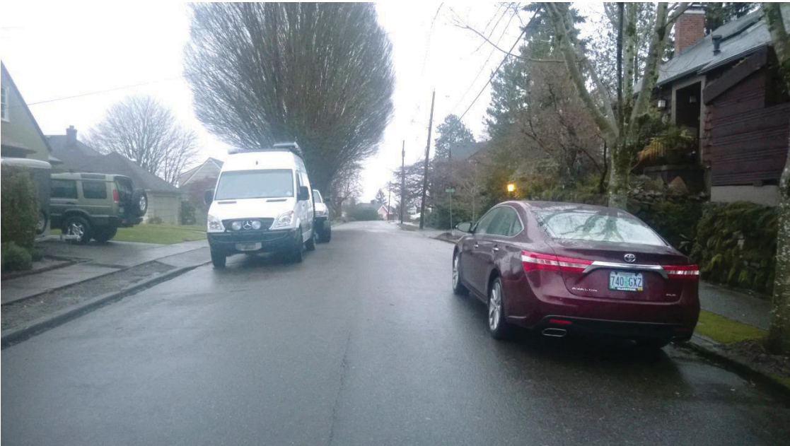
SW Evans, between SW 9 th and 10 th Avenues. One of the more improved roads in the area, however, due to the narrow road width, emergency vehicles can be limited by parked cars.
