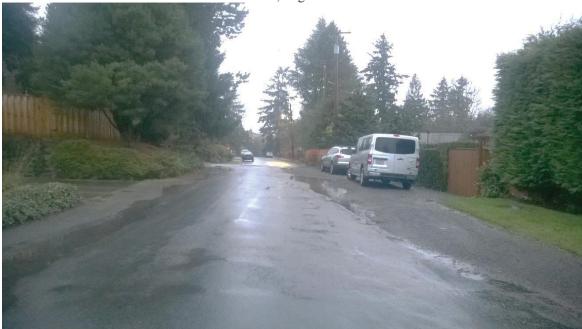
SW Hume Street, facing west at SW 11 th Avenue. Under-improved - lacking sidewalks, curbs and gutters.
