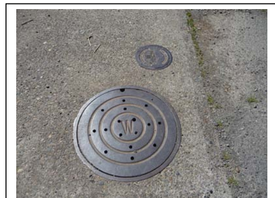
Figure 13. Manhole and CIV in road on Lincoln Drive
