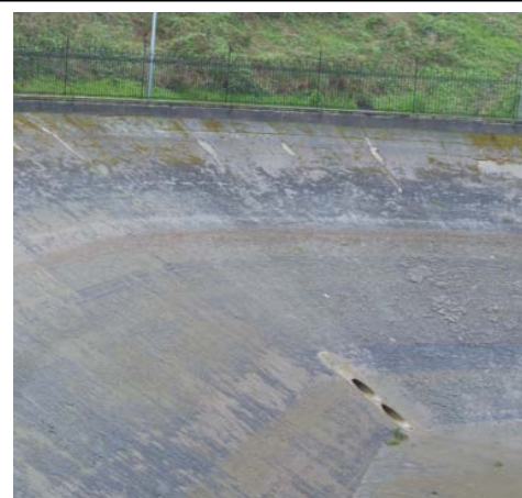
Figure 36. Openings in Reservoir 1 for the pipes connecting to Reservoir 5.
