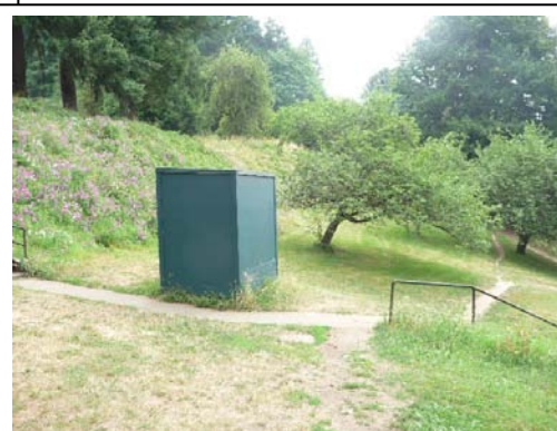
Figure 21. East access to Work Area 5 by stairs, hand rail and building.
