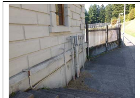
Figure 47. Gatehouse 6 East showing existing penetrations with condulets and conduits. Side view.
