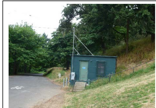
Figure 15. Existing building (identified as the 44-inch Meter House in the Park District nomination) by Southside Stairs
