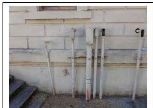
Figure 48. Gatehouse 6 East showing existing wall penetrations and conduits. Front view.
