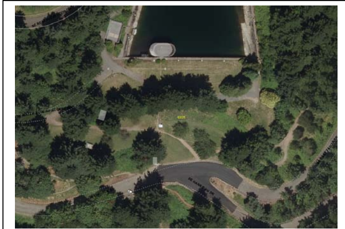
Fig. 17. Work Areas 4 and 5 showing road surface repair. Also shows area of “Terrace Garden” (discussed in WA 5 section, below).
