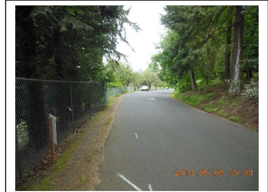
Figure 10. New 48-inch Pipe alignment at junction between Work Areas 2 and 3 in Lincoln Drive
