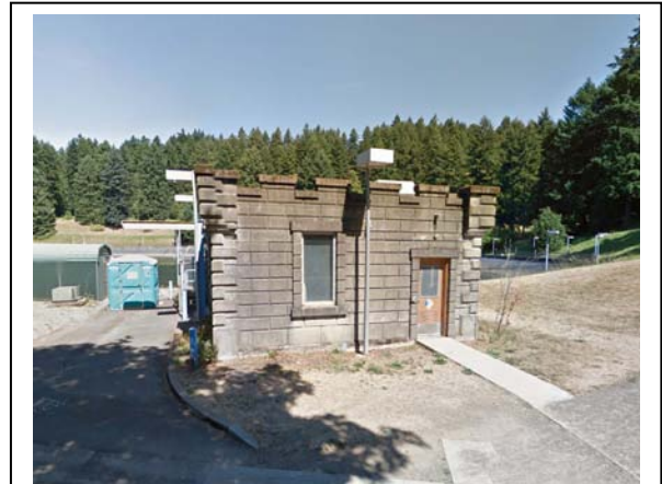
Figure 43. Weir building from the road facing the wall where the pipe enters the building. Photo from Google Street View (©2014 Google).
