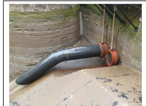
Figure 38. Two outlet pipes in south end of Reservoir 1 showing plastic
