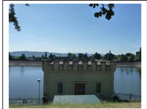
Figure 46. Gatehouse 6 East roof. Existing vent barely visible from Work Area 7.
