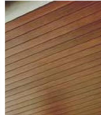
IPE PLANK SOFFIT AND PARTITION SCREEN
