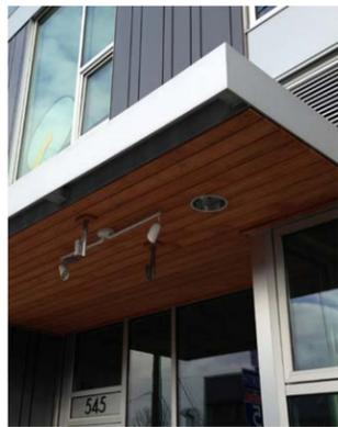
STEEL AWNING WITH IPE PLANK SOFFIT
