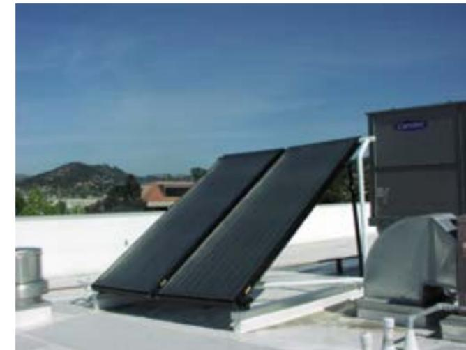
**ROOF MOUNTED SOLAR HOT WATER PANELS EXAMPLE**
