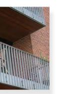
(05.63) Balcony Pipe Guardrails Galvanized Finish
