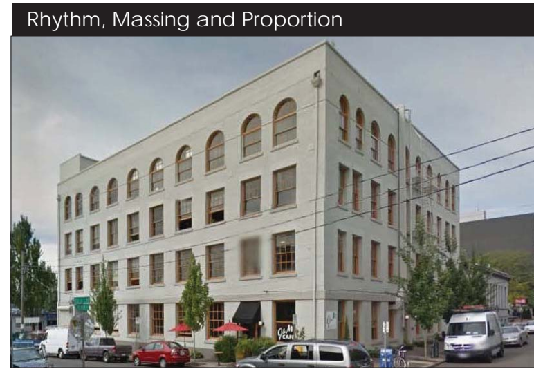
537 SE Ash Street
