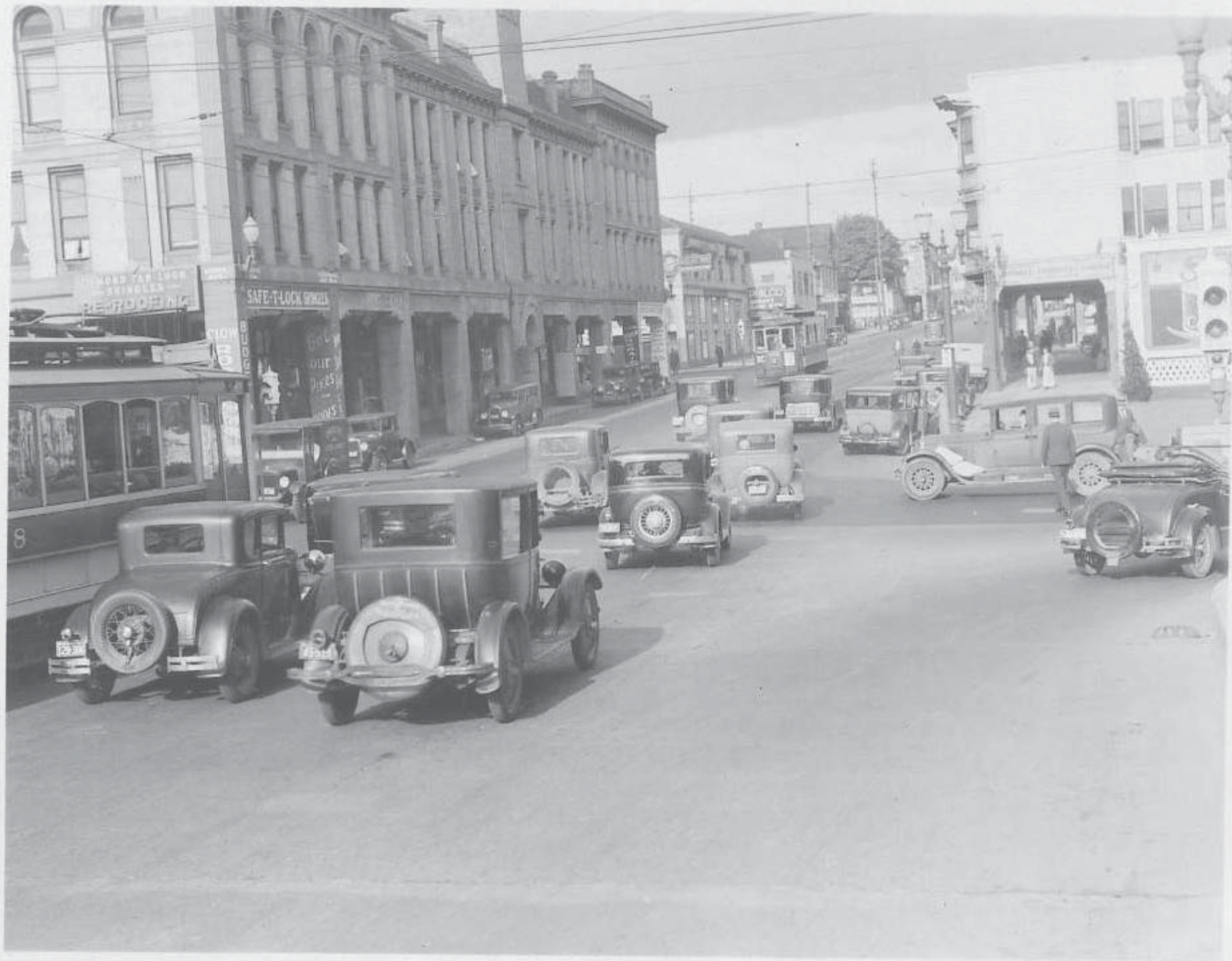
East approach of BURNSIDE BRIDGE. Showing arcaded structures.
