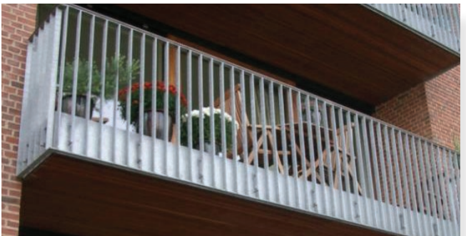
(05.63) Balcony Pipe Guardrails Galvanized Finish
