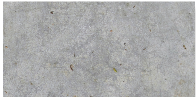
Cast In Place Concrete Base
