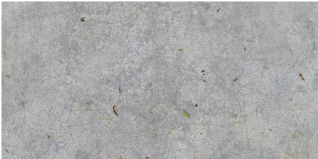
Cast In Place Concrete Base & Planter Walls
