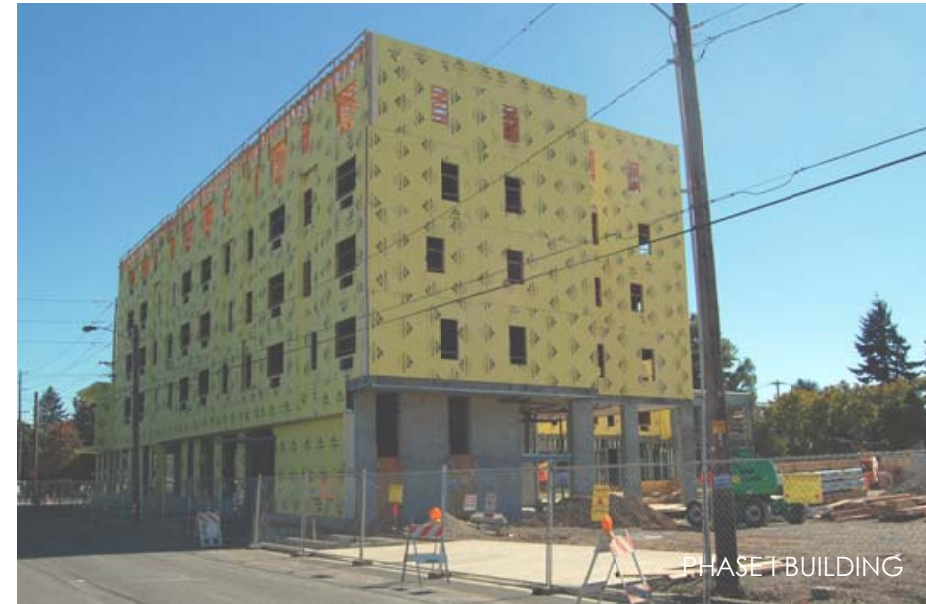
SW LOT ADJACENT TO PHASE II SITE & PHASE I BUILDING
