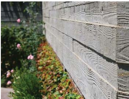
D STAINED CONCRETE CAST W/ BOARD FORM LINER
