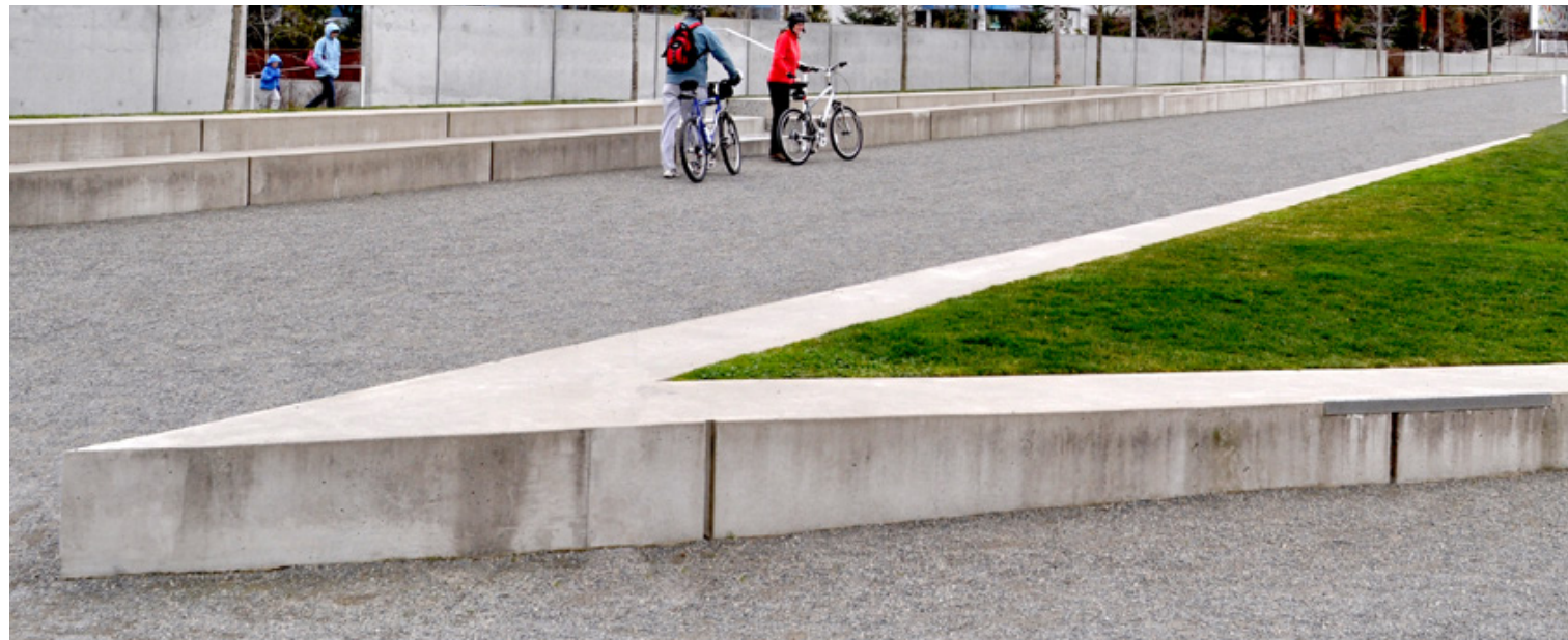
ANGULAR CONCRETE SEATWALL / PLANTER
