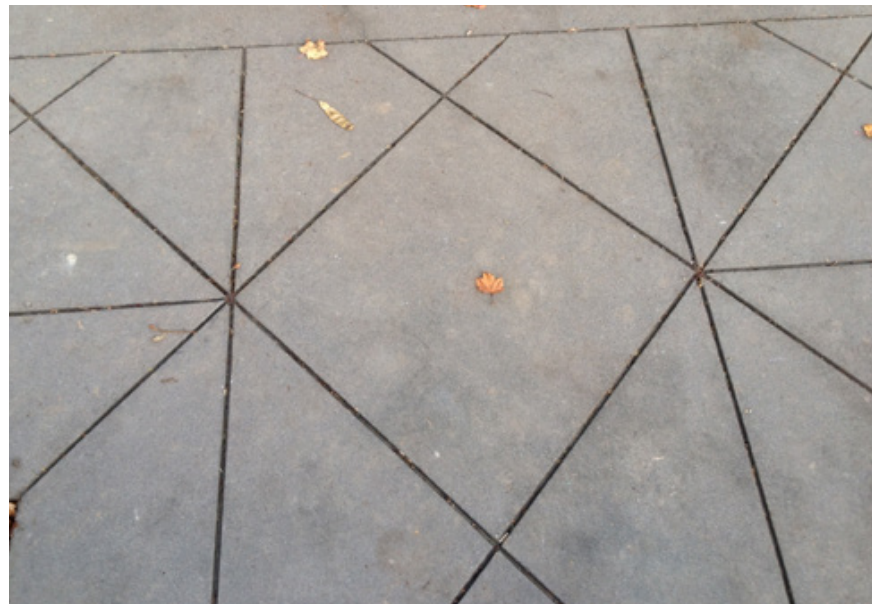
DIAGONALLY SCORED CONCRETE
