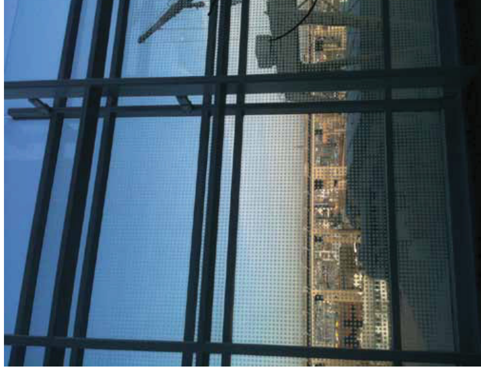
View of fritted window pattern (above) at the OHSU Center for Health and Healing demonstrate how frit patterns can be designed to afford views out (Photo at left is a close-up). Frits can synergistically reduce solar heat gain, afford privacy, and provide visual cues to approaching birds. No collisions have been documented at this building in four seasons of monitoring. Photo: Mary Coolidge
