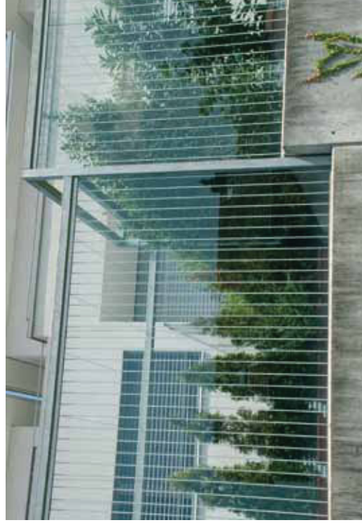
The white stripes on this glass wall are an easy way to make a very dangerous area safe for birds. Photo: Hans Schmid
