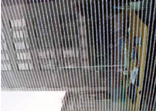
The glass facade of SUVA Haus in Basel, Switzerland, renovated by Herzog and de Meuron, is screen-printed on the outside with the name of the building owner. Photo: Miguel Marqués Ferrer
