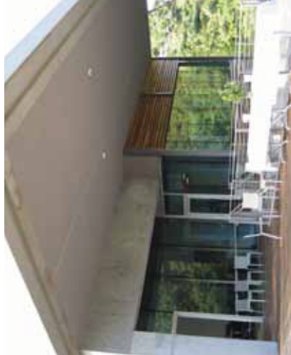
Overhangs block viewing of glass from some angles, but do not necessarily eliminate all reflections. Photo: Christine Sheppard, ABC
