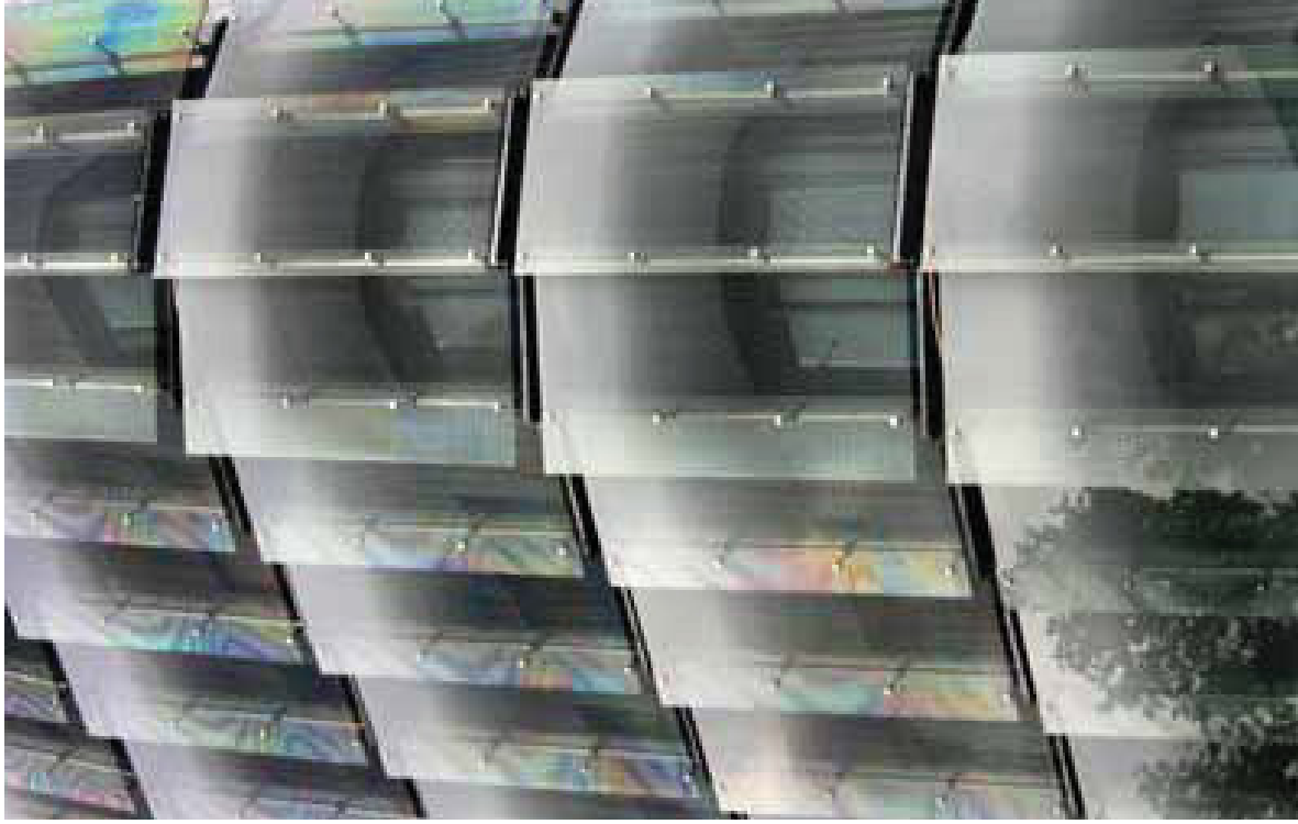
Galeo, part of a complex designed by Atelier Christian de Portzamparc in Issy les Moulineaux, France, has an external skin of printed glass scales which help to reduce reflections. Photo: Sipane
