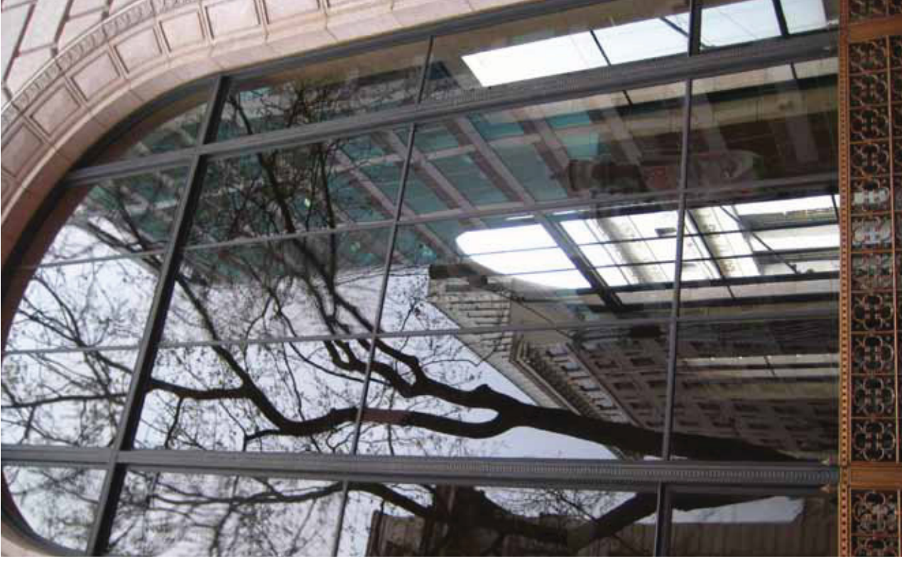
The mirrored windows at Lewis and Clark were highly reflective on gray days as well sunny days. Photo: Mary Coolidge
