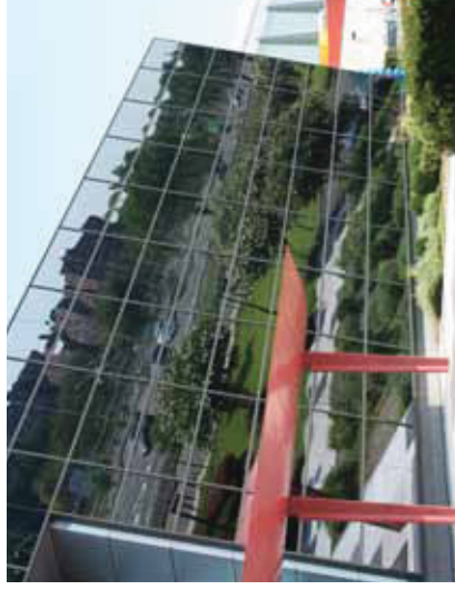
The angle on the New York Times printing plant facade is not sufficient to eliminate deceptive reflections of nearby vegetation. Photo: Christine Sheppard, ABC
