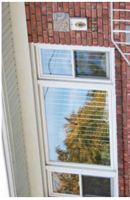
Reflections on home windows are a significant source of bird mortality. Partially opened vertical blinds may break up reflections enough to reduce the hazard to birds. Photo: Christine Sheppard, ABC
