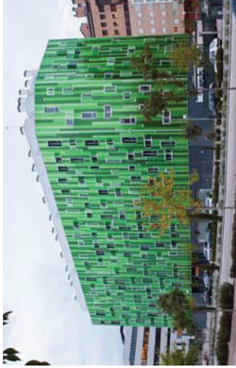
Madrid's Vallecas 51, designed by Somos Arquitectos, uses open-celled polycarbonate panels – a sustainable and recyclable skin that presents no threat to birds. Photo: Victor Tropchenko
