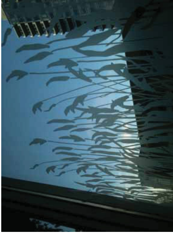
Privacy film on Mirabella windows preserves light entry and views out while marking the window for birds. Such film is more effective if applied to the exterior. Photo: Mary Coolidge
