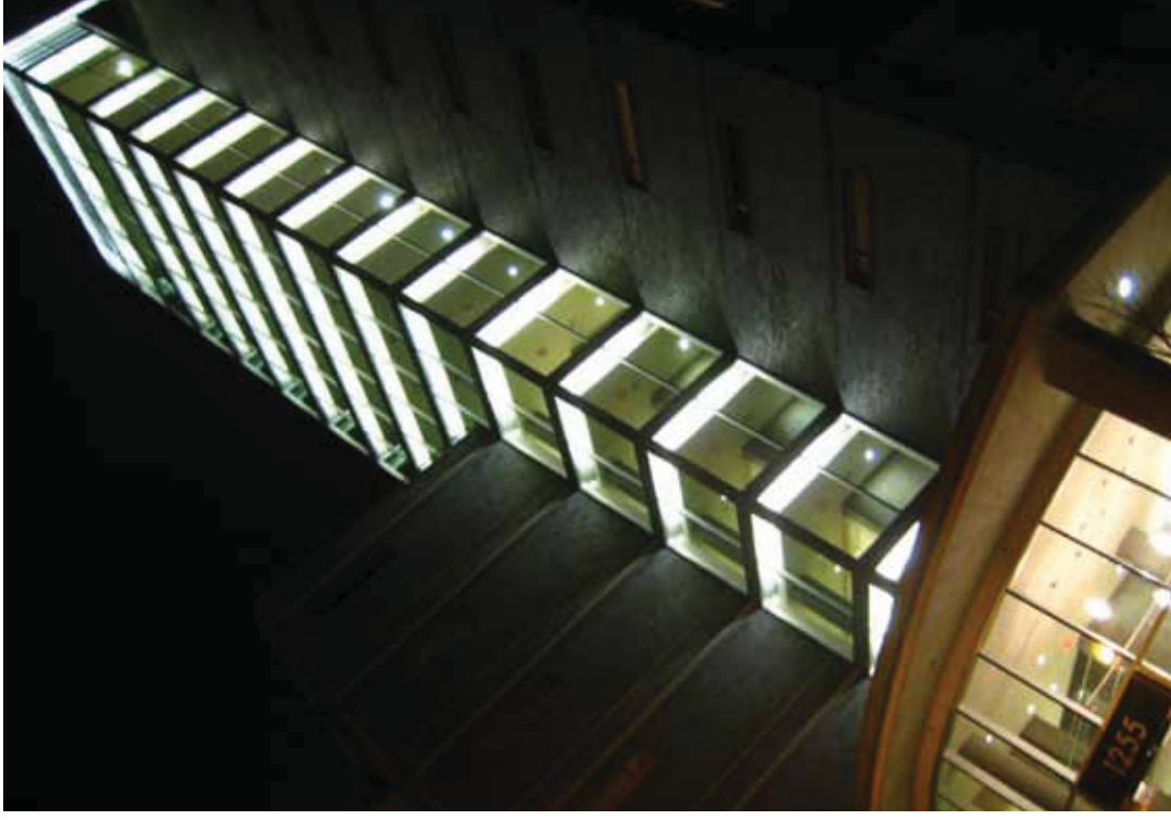
Light spill is apparent from this stairwell in the Pearl District, and could be minimized by exterior shielding. Photo: Mary Coolidge
