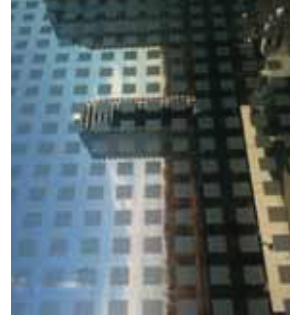
View of fritted window pattern (above) at the OHSU Center for Health and Healing demonstrate how frit patterns can be designed to afford views out (Photo at left is a close-up). Frits can synergistically reduce solar heat gain, afford privacy, and provide visual cues to approaching birds. No collisions have been documented at this building in four seasons of monitoring. Photo: Mary Coolidge
