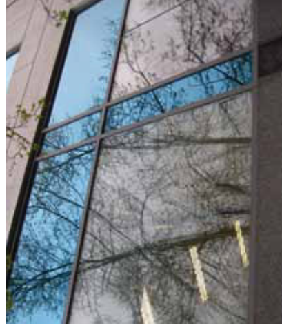
Tinted windows at the State Building readily reflect vegetation. More testing on colors and density is needed. Photo: Mary Coolidge
