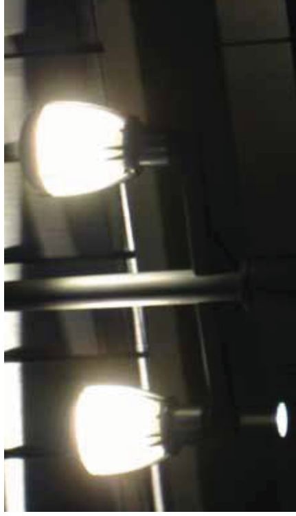
Though newer acorn-style light fixtures in South Waterfront have incorporated some shielding design, full cut-off improvements to the design of these fixtures would reduce contribution to light pollution. Photo: Mary Coolidge
