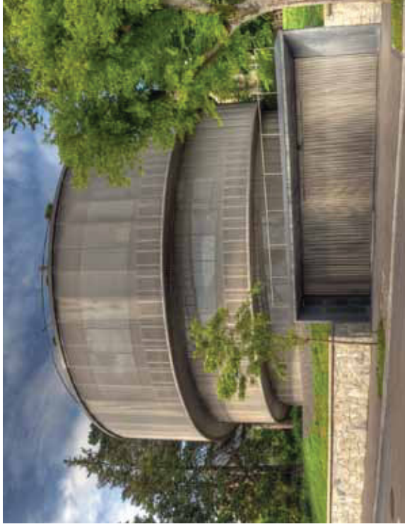
The steel mesh enveloping Zurich's Cocoon in Switzerland, designed by Camenzind Evolution Ltd, provides privacy and protects birds, but still permits occupants to see out. Photo: Anton Volgger
