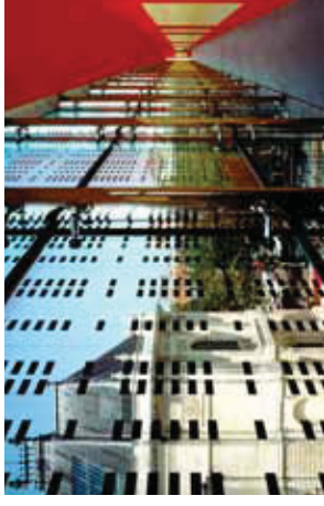
External frit, as seen here on the Life Museum of Fine Arts, by Iboos and Vitart, is more effective at breaking up reflections than patterns on the inside of the glass. Photo: G. Fessy
