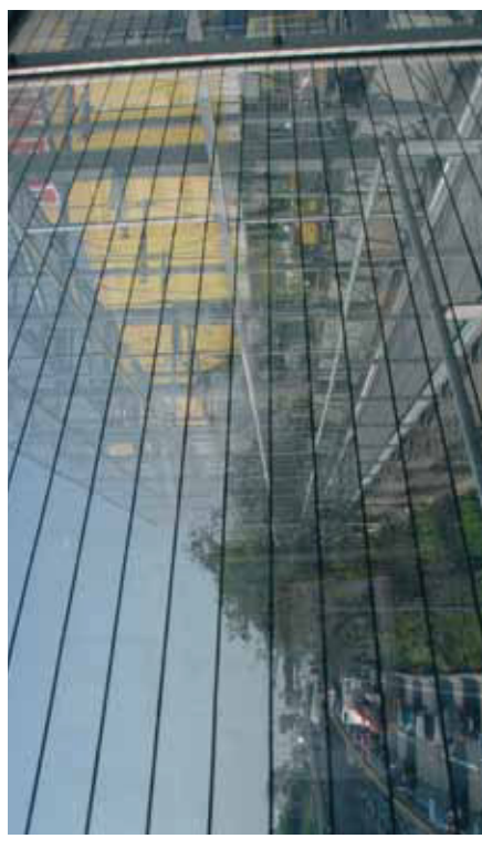
A pattern of narrow horizontal stripes has proven to be highly effective at deterring bird collisions, while covering only about 7% of the surface of the glass. Photo: Hans Schmid
