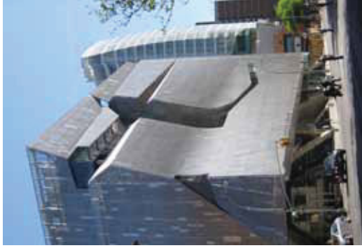
41 Cooper Square in New York City, by Morphosis Architects, features a skin of perforated steel panels fronting a glass/aluminum window wall. The panels reduce heat gain in summer and add insulation in winter while also making the building safer for birds. Photo: Christine Sheppard, ABC
