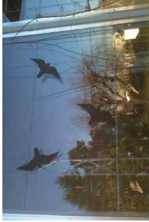
Silhouettes placed every 12 inches on the exterior of this residential window are spaced too far apart to reliably eliminate all strikes, but will likely reduce strike incidence.
