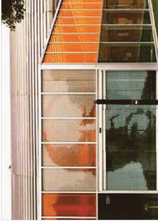
The IIT Student Center in Chicago uses faceted glass. Panelite panels and a dot matrix pattern (above) in its facade. These elements create visual noise which is perceptible to birds.
