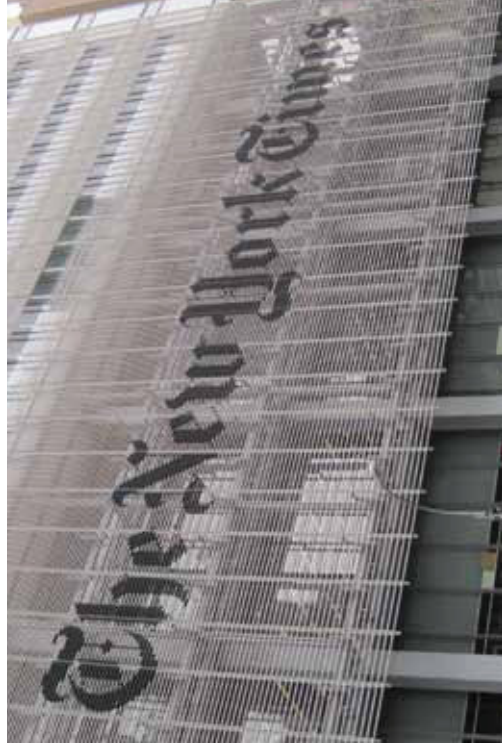
The façade of the New York Times building, by FX Fowle and Renzo Piano, is composed of ceramic rods, spaced to let occupants see out, while minimizing the extent of exposed glass. Photo: Christine Sheppard, ABC
