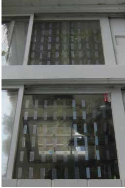
Tape decals (Window Alert shown here) placed following the 2 x 4 rule can be effective at deterring collisions. Photo: Christine Sheppard, ABC
