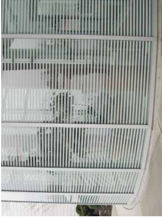
Dense stripes of internal frit on University Hospital's Twinsburg Health Center in Cleveland, by Westlake, Reed, Leskosky will overcome virtually all reflections. Photo: Christine Sheppard, ABC
