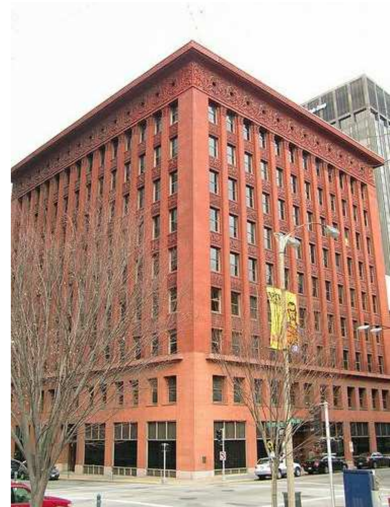
WAINWRIGHT BUILDING - SULLIVAN
