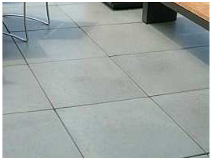
A. SCORED CONCRETE PAVING W/ SAND FINISH
