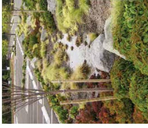
Native plantings in a meandering vegetated swale could function as an urban stream to manage stormwater and treat roadway runoff.
