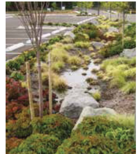
Native plantings in a meandering vegetated swale could function as an urban stream to manage stormwater and treat roadway runoff.
