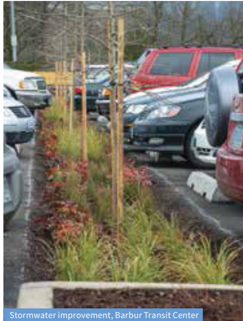
Stormwater improvement, Barbur Transit Center
