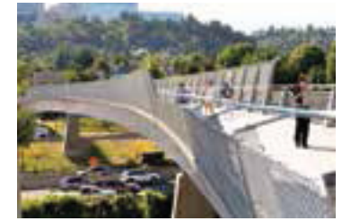
Darlene Hooley pedestrian bridge at Gibbs Street.
