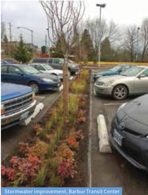
Stormwater improvement, Barbur Transit Center
