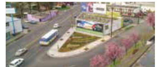
Stormwater facility on Sandy Blvd.
