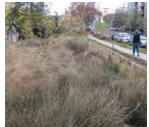
Stormwater infiltration facilities in excess rights of way.
