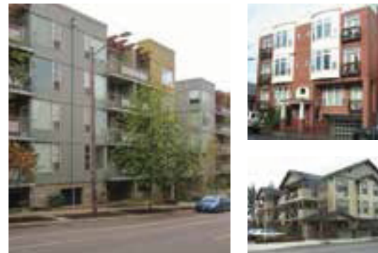
Low-profile, higher density housing options can be provided in a variety of arrangements.
