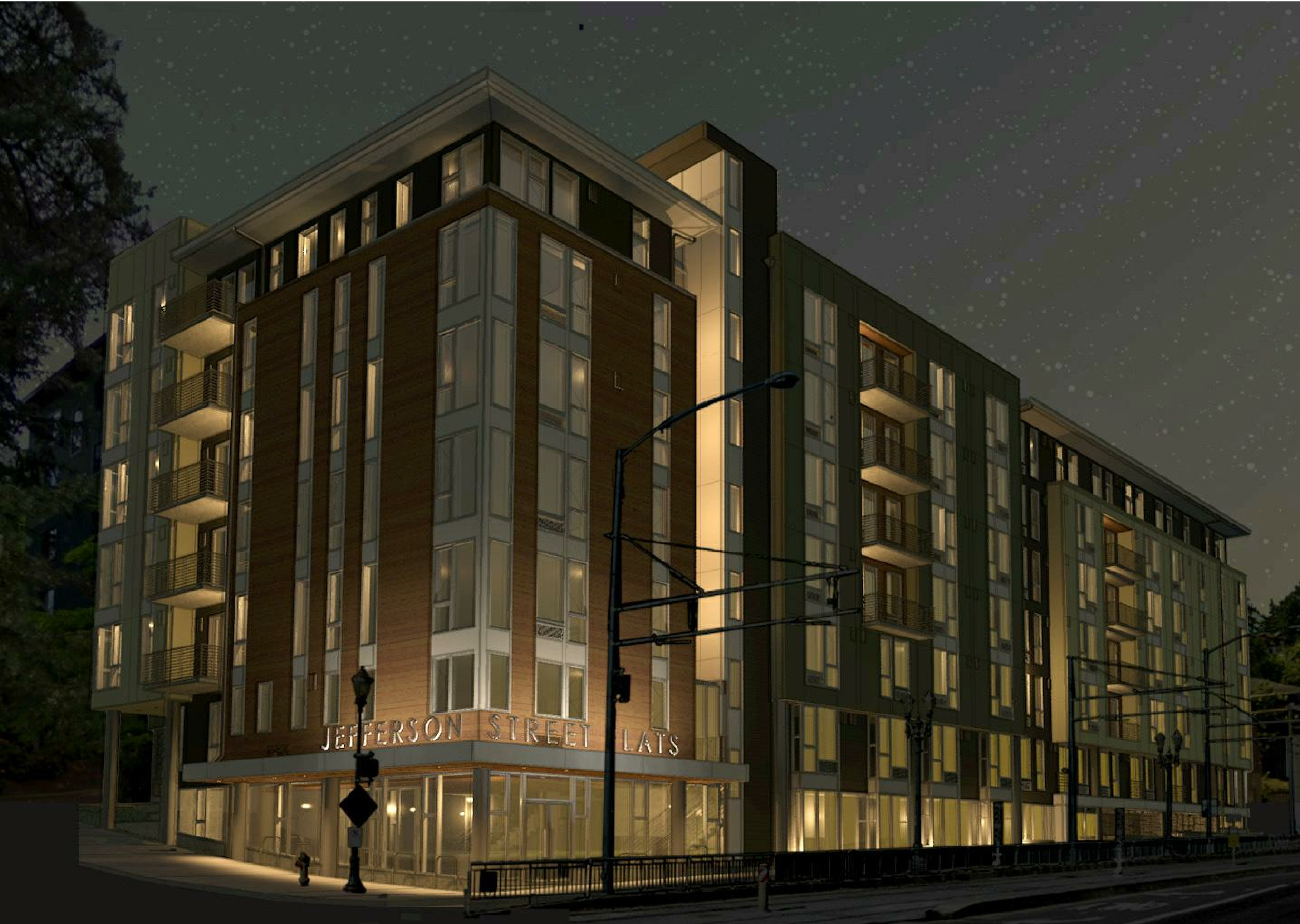
NIGHT VIEW - NE CORNER OF BUILDING
