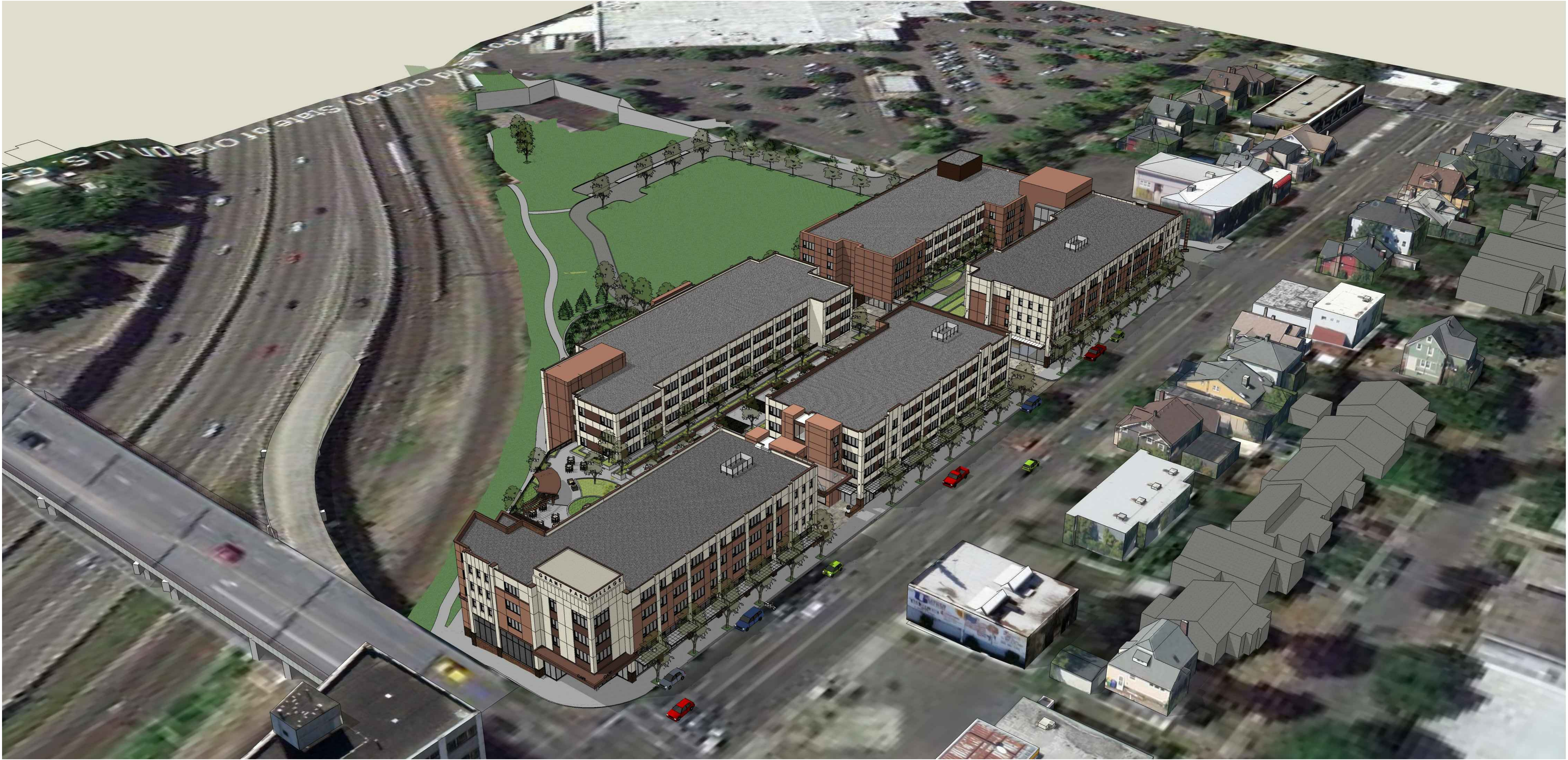
AERIAL VIEW FROM NORTHEAST
