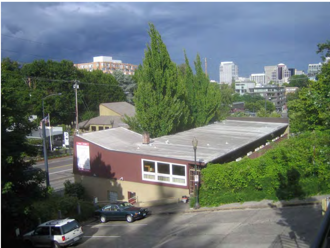
WEST ON 21 ST SHOWING EXISTING BUILDING
