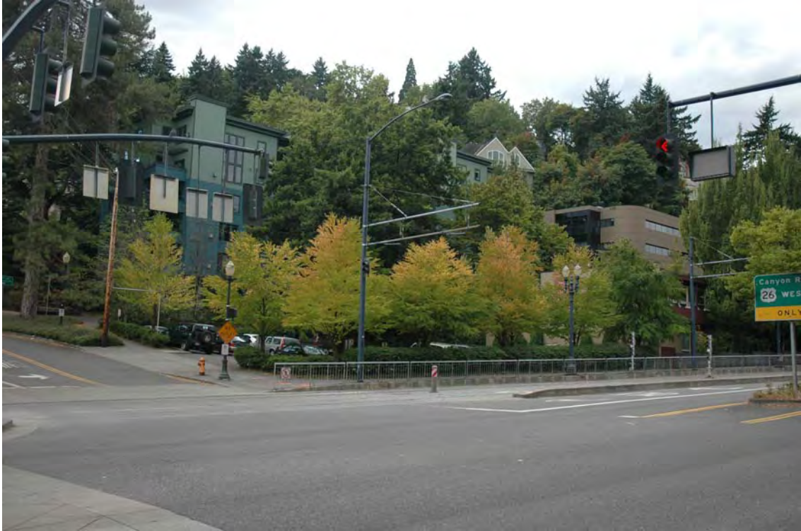
NE CORNER SHOWING MAX LIGHT RAIL LINE AND ARBOR VISTA
