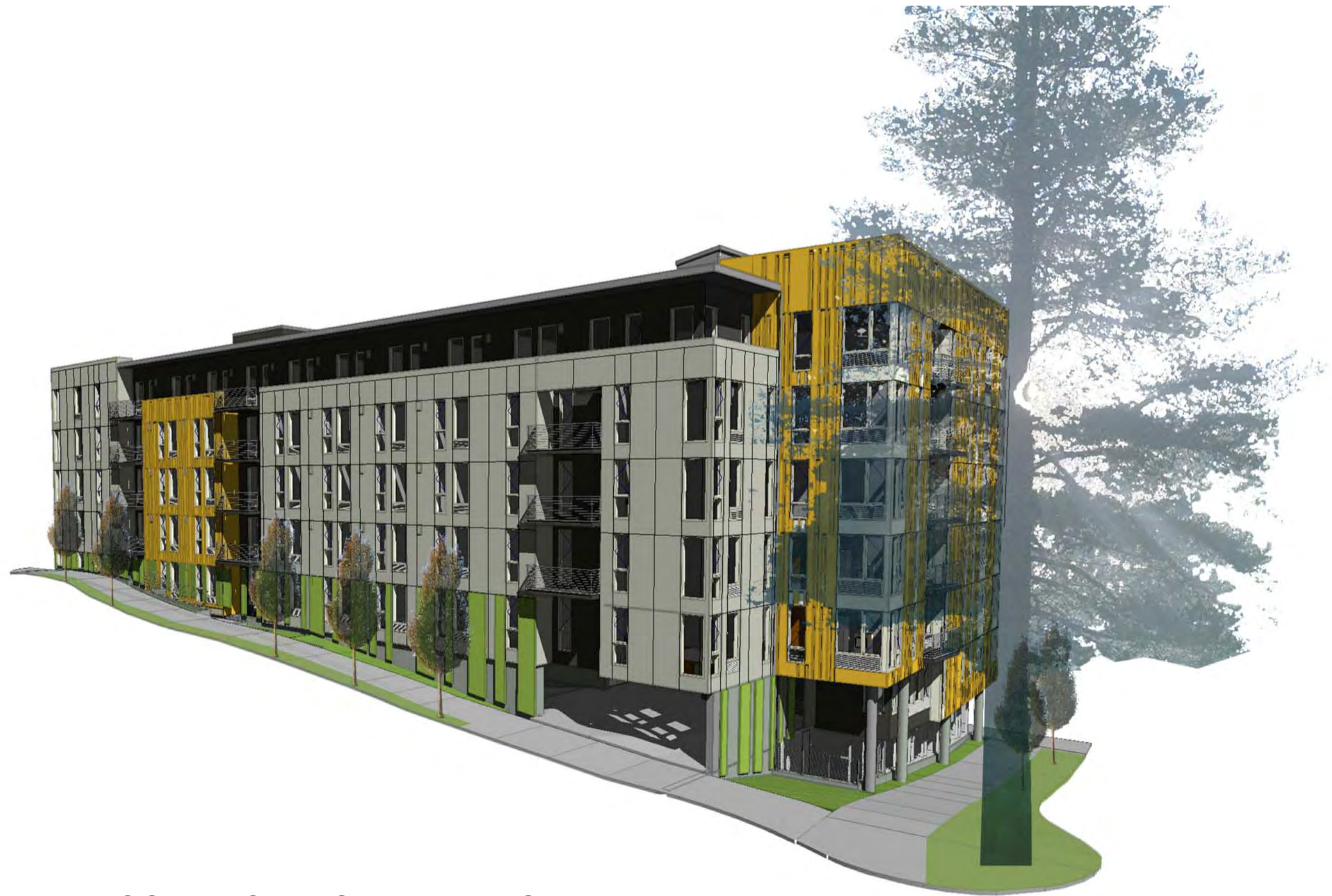
VIEW - SOUTH SIDE OF BUILDING
