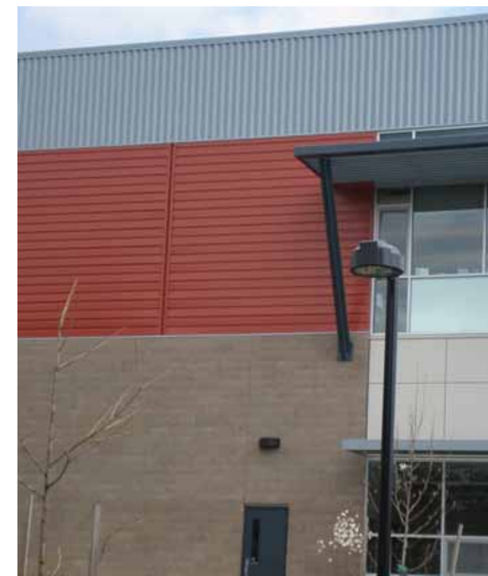
BONNY SLOPE SCHOOL, PORTLAND - USED CS-620, FORMABOND PANELS, & STYLE-RIB
