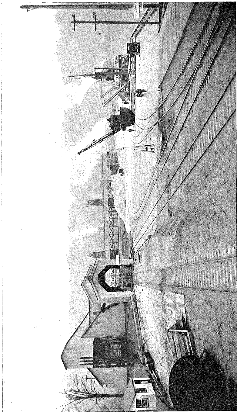
PIER NO. 5 WITH BULK STORAGE PLANT, MUNICIPAL TERMINAL NO. 4. THE VIEW IS TOWARD THE HARBOR WITH SLIP NO. 3 TO THE RIGHT, SULPHUR CARGO BEING DISCHARGED ON THE PIER BY LOCOMOTIVE CRANE WITH CLAM SHELL BUCKET
