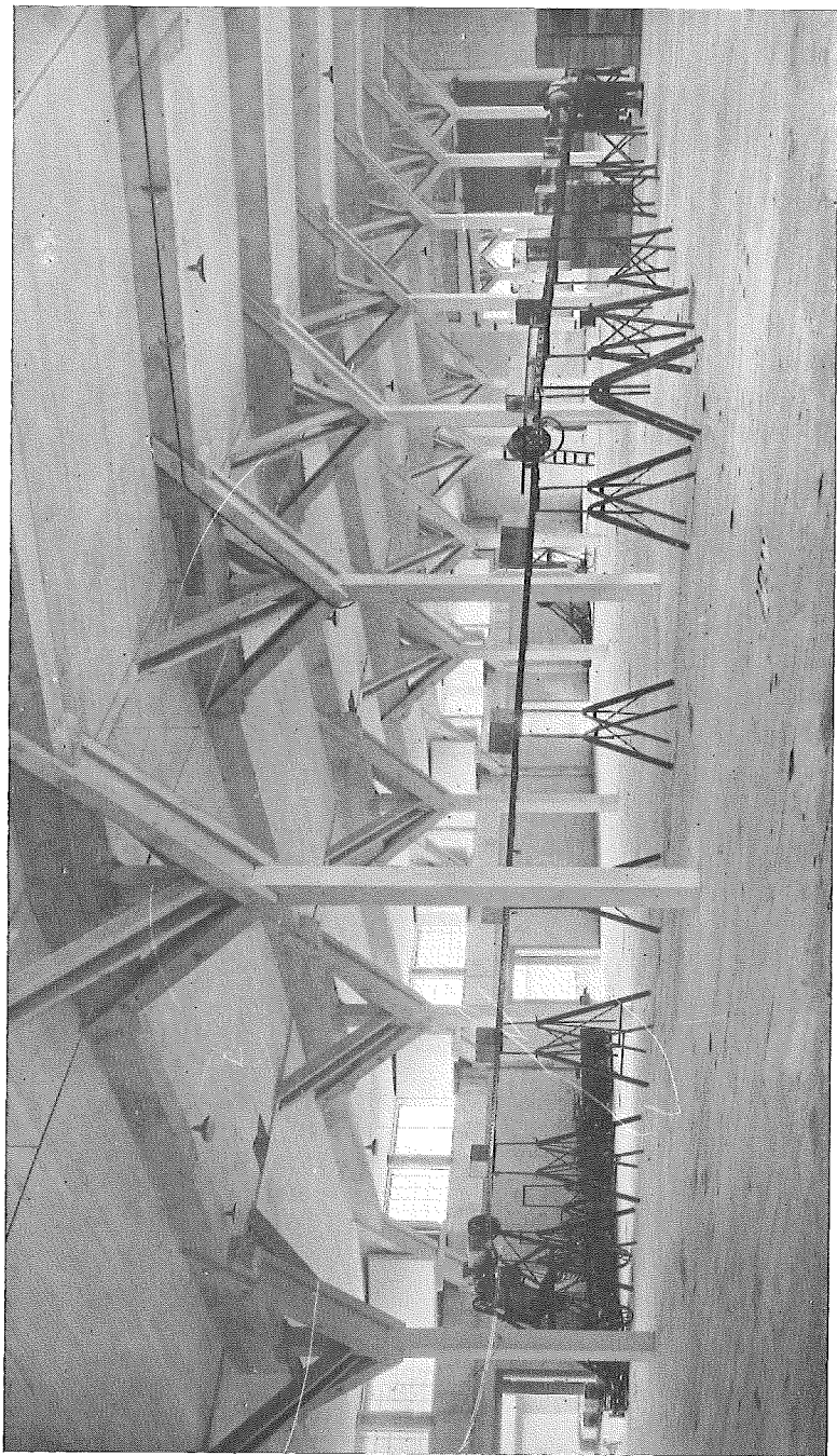
INTERIOR VENTILATED WAREHOUSE FOR APPLE STORAGE, MUNICIPAL TERMINAL NO. 4. COMPLETE POWER AND GRAVITY CONVEYOR SYSTEMS ARE PROVIDED FOR ECONOMICAL HANDLING
