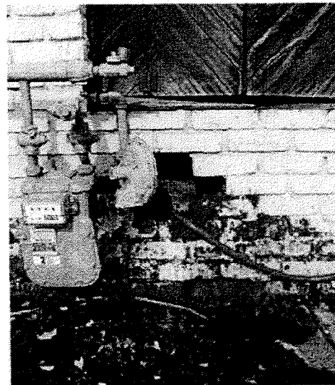
existing conditions at ground
