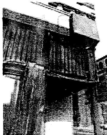
existing facade & walkway at entry
