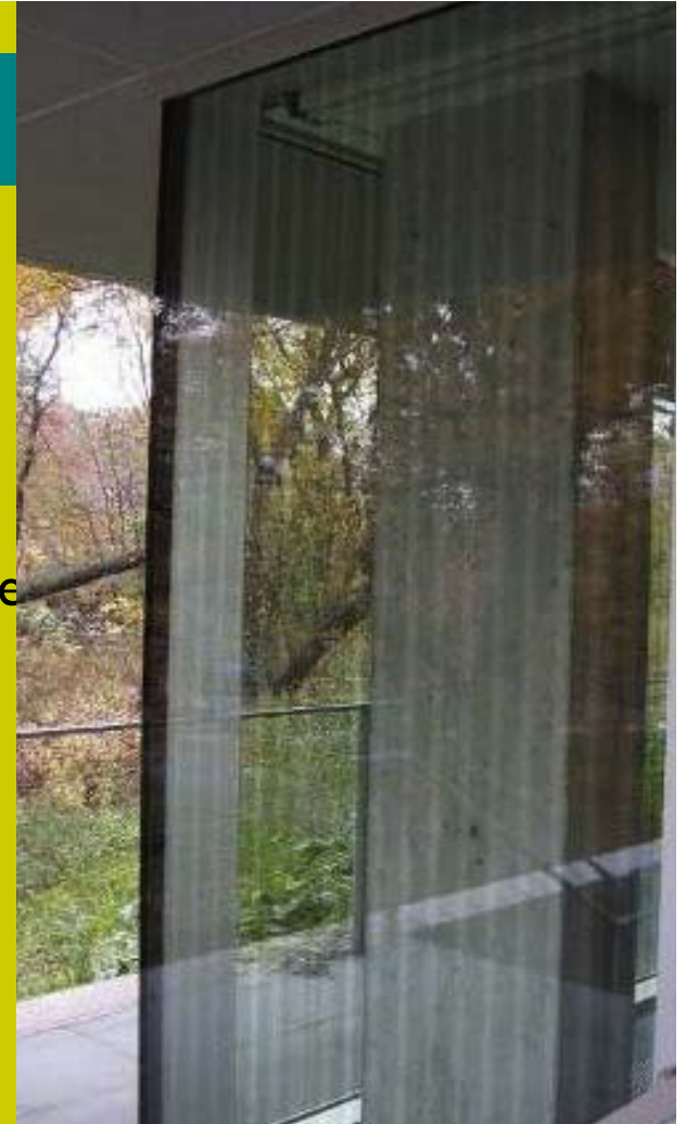
Bird-friendly glass on corner windows at WCS, Bronx Zoo
