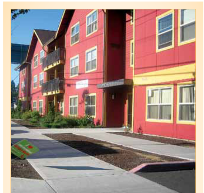
Leander Court, an attractive multifamily housing complex near SE 122nd and Holgate.
