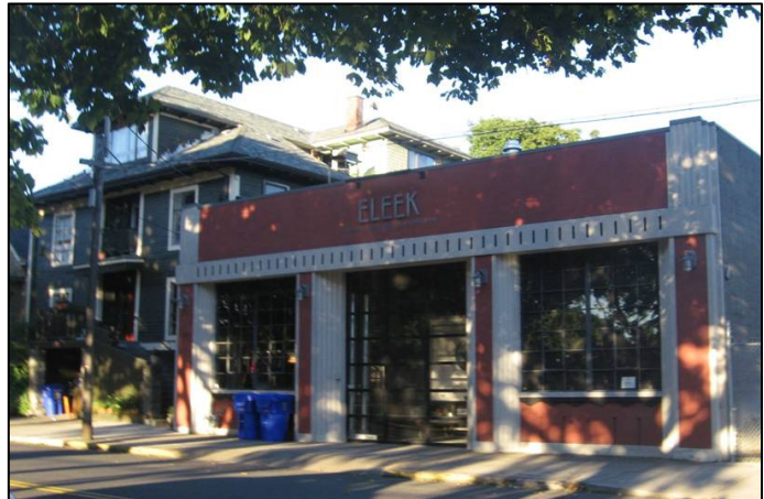
Commercial uses along N Flint
