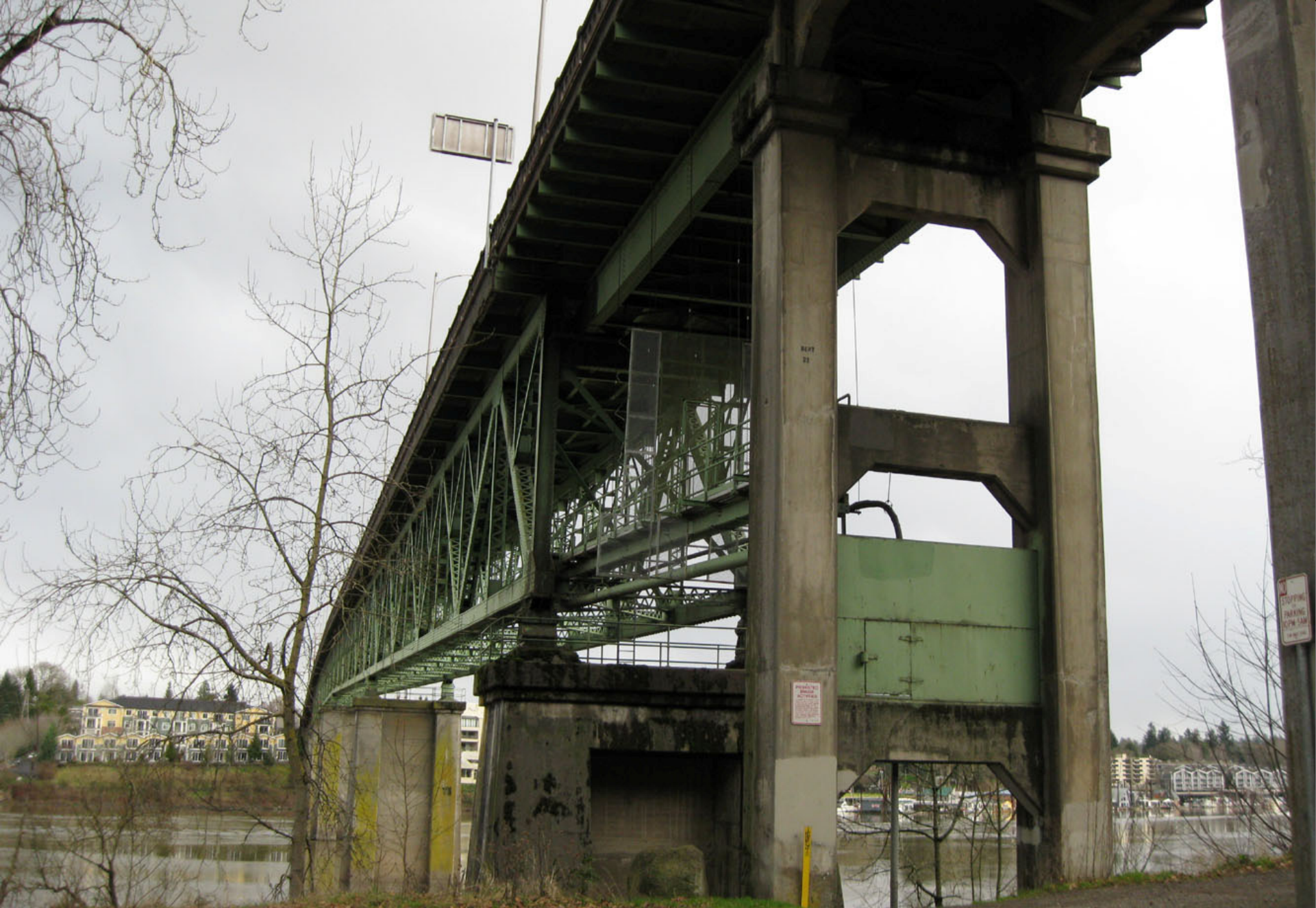
Sellwood Bridge supports at Powers Marine Park
