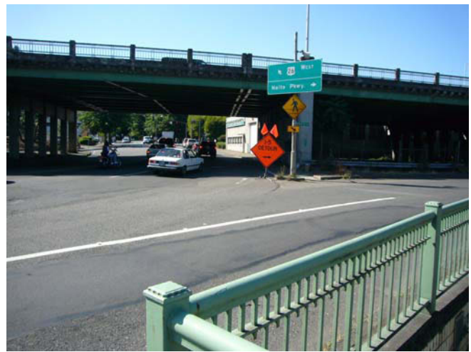
Looking west down Kelly Avenue from NE tunnel entrance.
