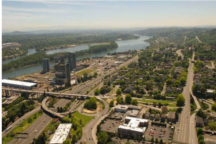
This photograph shows the ramps at the west end of the Ross Island Bridge - looking southbound.
