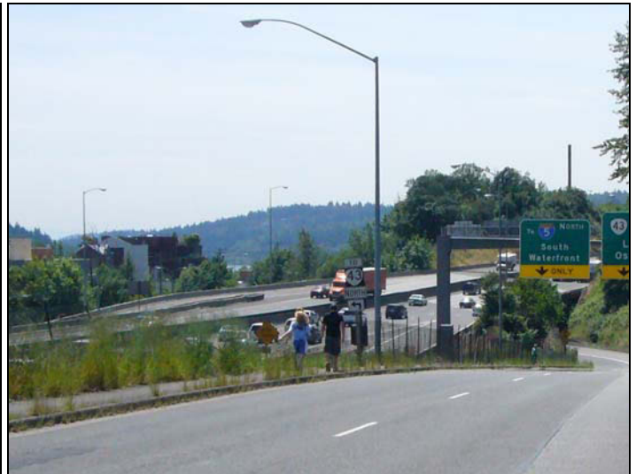
Sidewalk along west side of SW Hood Avenue, leading to I-5 underpass – jersey barriers recommended to be placed between roadway and sidewalk
