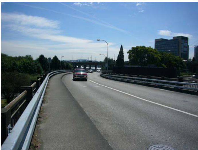
Sidewalk (5.5 feet) on north side of Macadam/City Center Ramp looking east with South Waterfront District development in the background.
