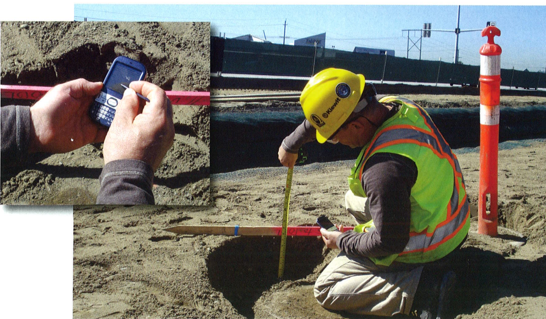
Mobile Information Collection for Kiewit, or "MICK," coupled with Centric Project brings Kiewit ever closer to the goal of recording project data and quantities electronically with the data available to all system users on a realtime basis.
