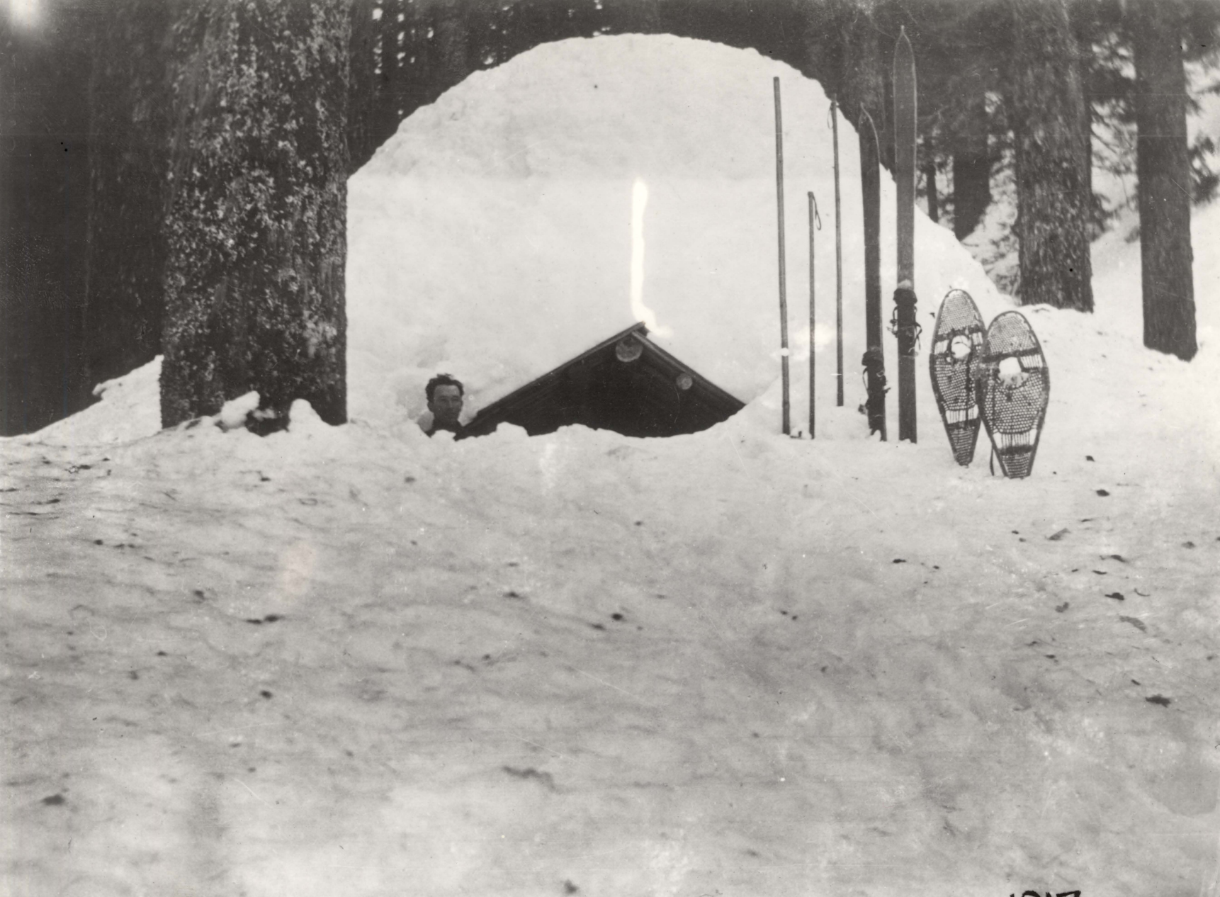
Water Department Cabin, Bull Run Lake, April 5, 1917.
