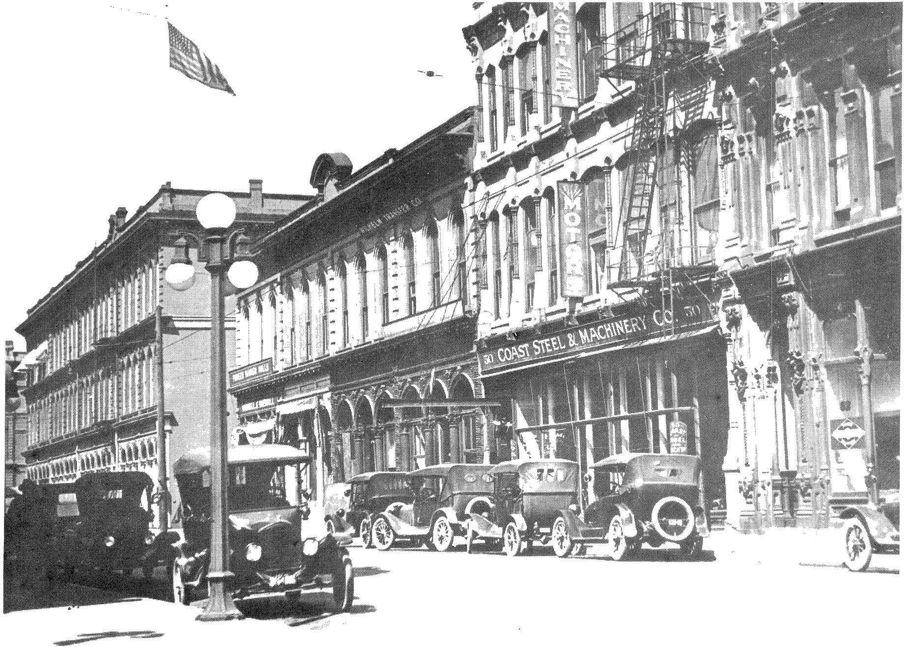
First Avenue in the 1920s. A modified version of the street light is proposed as the design standard for the District
