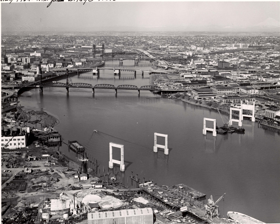
May 1964 - Marquam Bridge Piers
