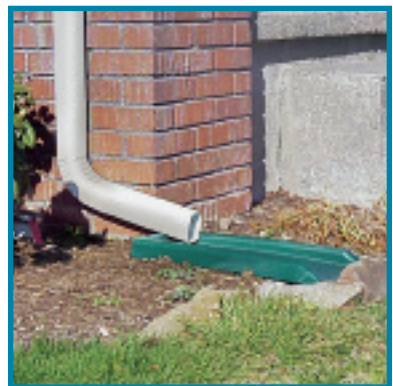
▲ Disconnected downspout
