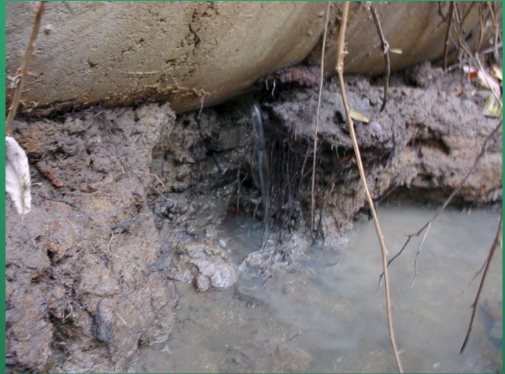
Sanitary pipe leaking directly into Stephens Creek
