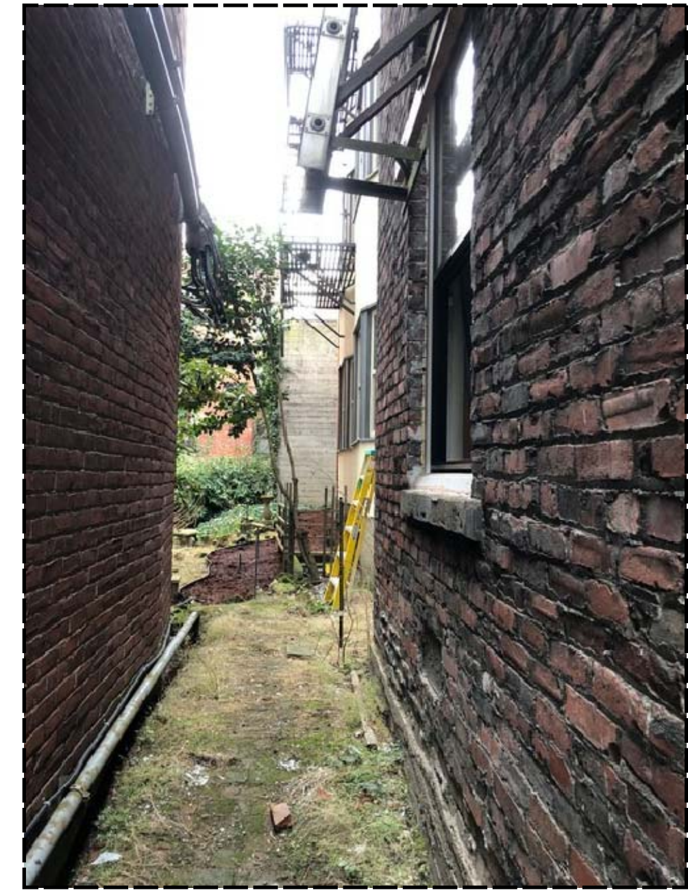
TYPICAL EGRESS WINDOW @ EAST SIDE OF BUILDING, EGRESS PATH TO TRINITY PLACE LEFT AT CORNER OF ADJACENT BUILDING.
