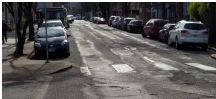
Portland road in poor pavement condition
