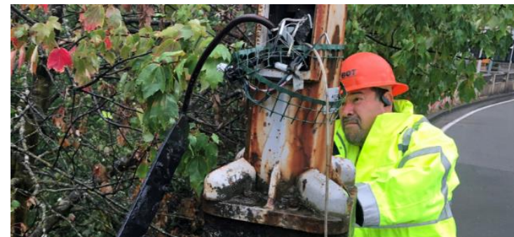
Vandalism repair of a streetlight
