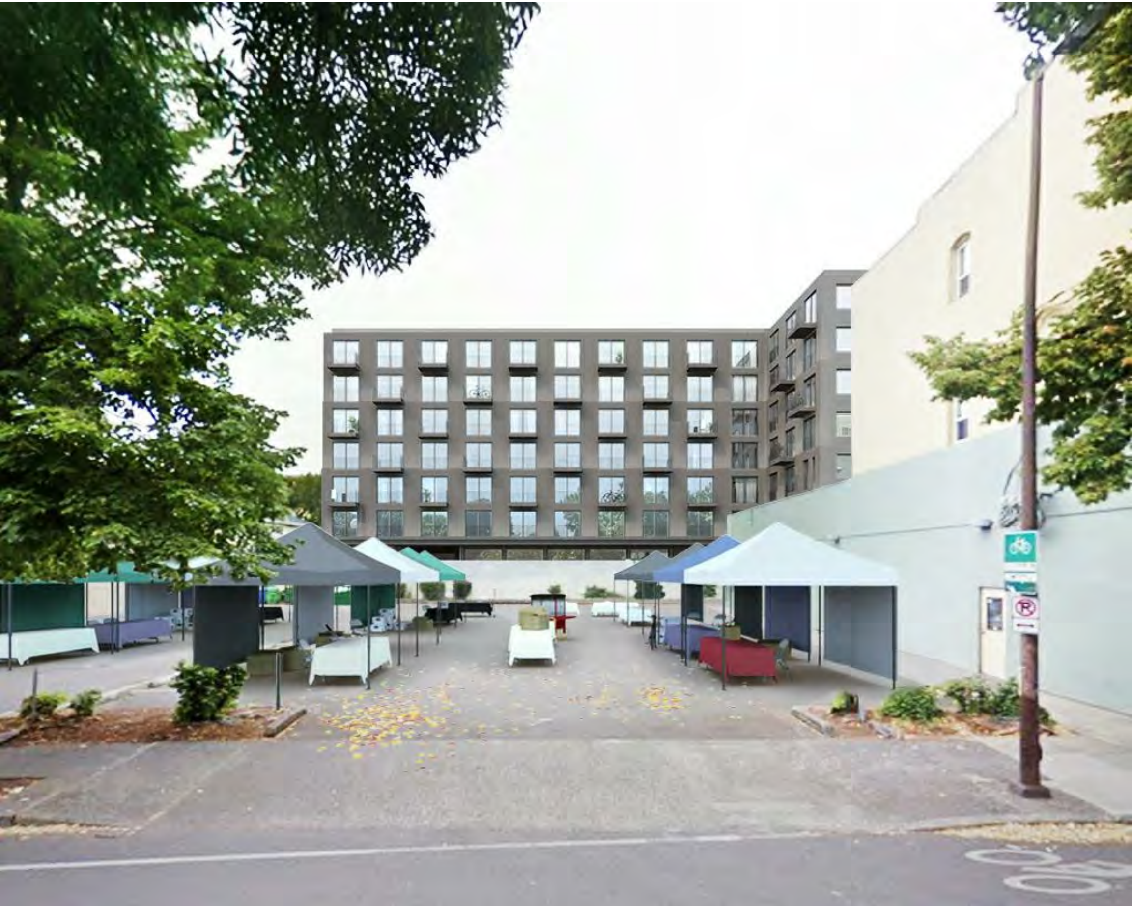
Exterior view from the Urban League parking lot
