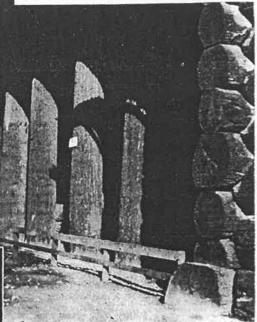
ENOUGH TIMBER for a small bungalow in almost every timber, this 'World's largest' log cabin, the Forestry building, looms huge compared with the figures of a service man and his companion standing at the foot of a 54-foot upright timbers supporting the center section.
