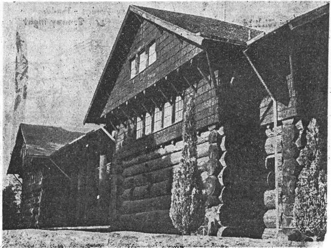
Settling side walls, which have twisted roof and balconies, dry rot and the general debilities of age have taken heavy toll of Forestry building, called the "biggest log cabin in the world."
