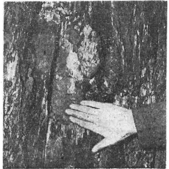
Dry rot has eaten into 44 bark-covered six-foot tree trunks which support sagging roof.
