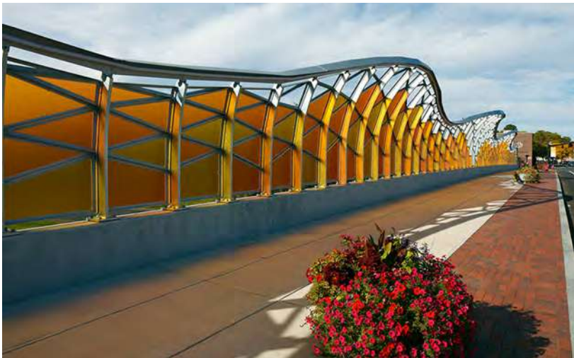
Acrylic panels on Beehive Bridge in New Britain, CT
